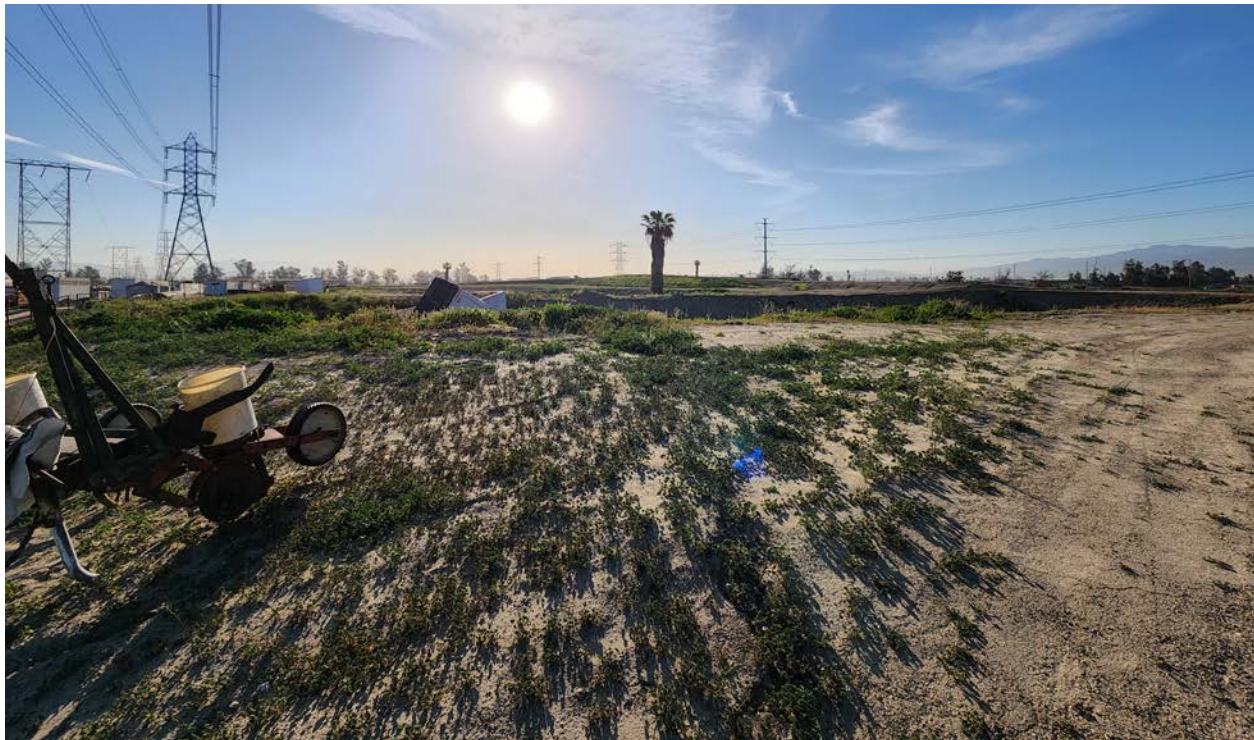
Photograph No. 4: Current site conditions at large southeastern berm, facing southeast.
