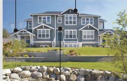
Blended wood clapboard siding, or shingles, and stucco
