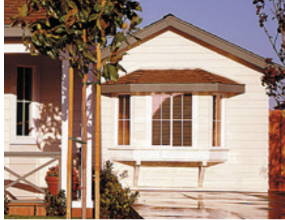
MULTI-PANE BAY WINDOW HORIZONTAL LAPPED SIDING
