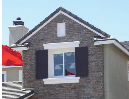
BRICK SIDING AND VERTICAL MULTI-PANED WINDOWS
