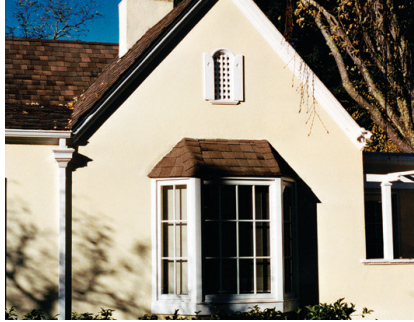
FEATURE WINDOWS & GABLE ACCENTS
