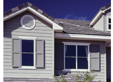
VENTED GABLE AND HORIZONTAL SIDING
