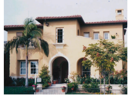
STUCCO WALLS WITH ARCHED OPENINGS
