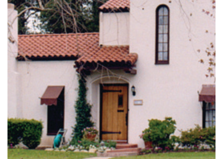
WELL ARTICULATED ENTRY
