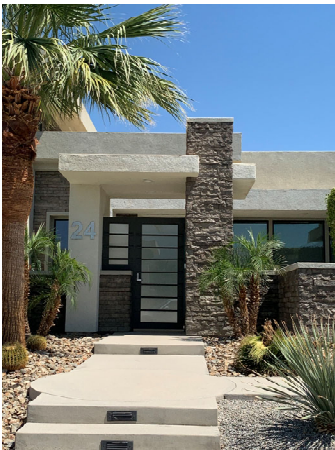
Low-pitched roofs behind a parapet
