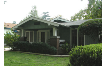
Entry door with side lights, shingle siding and wood posts with brick bases.
