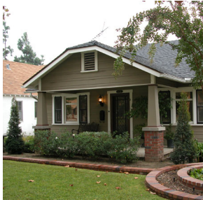
Covered porch with distinctive gable end treatment.
