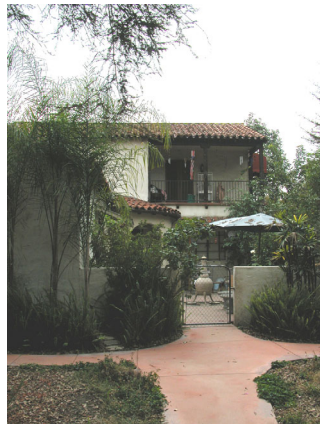
Heavy timber Deck Overlooking Entry Courtyard below
