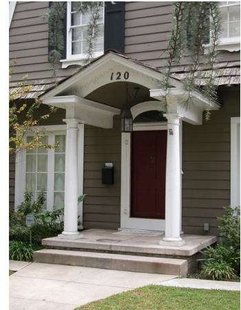
Paneled front door with arched transom above, classical columns supporting gabled porch roof.
