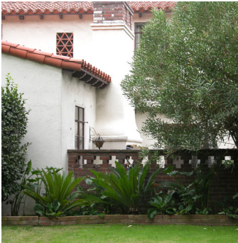
"S" tile roof with open eaves accentuated by decorative eave treatment and tile venting.
