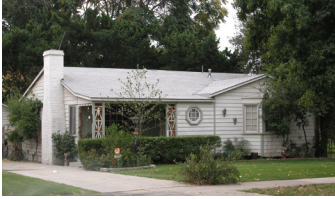
Long horizontal gable roof, with extensive use of lap siding and brick accent at chimney.
