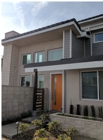
Entry porch with accent color door and metal column support.
