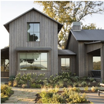
Simple well-proportioned windows.
