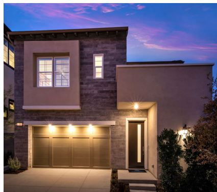
Contrasting materials and textures for various massing elements
