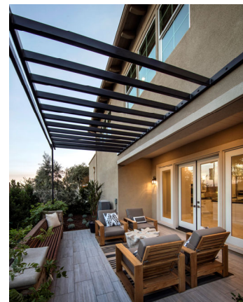
Porch with simple metal detailing.
