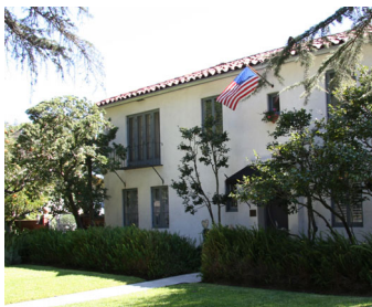
Simple Massing with Modest Wrought Iron Accents at Balcony and entry Awnings.
