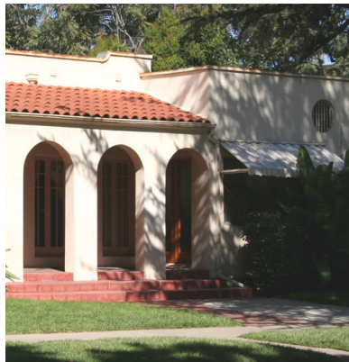
Arched recessed porch and shaped parapets.
