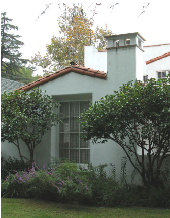
Tight rake with no exposed fascia, recessed feature window and decorative chimney cap.
