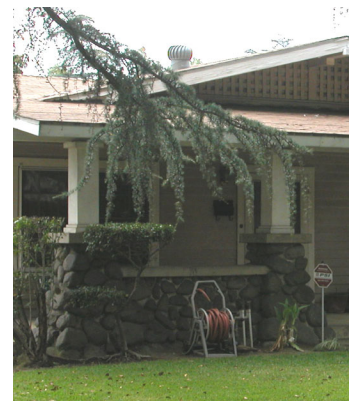
Exposed wood columns with battered stone base at porch.
