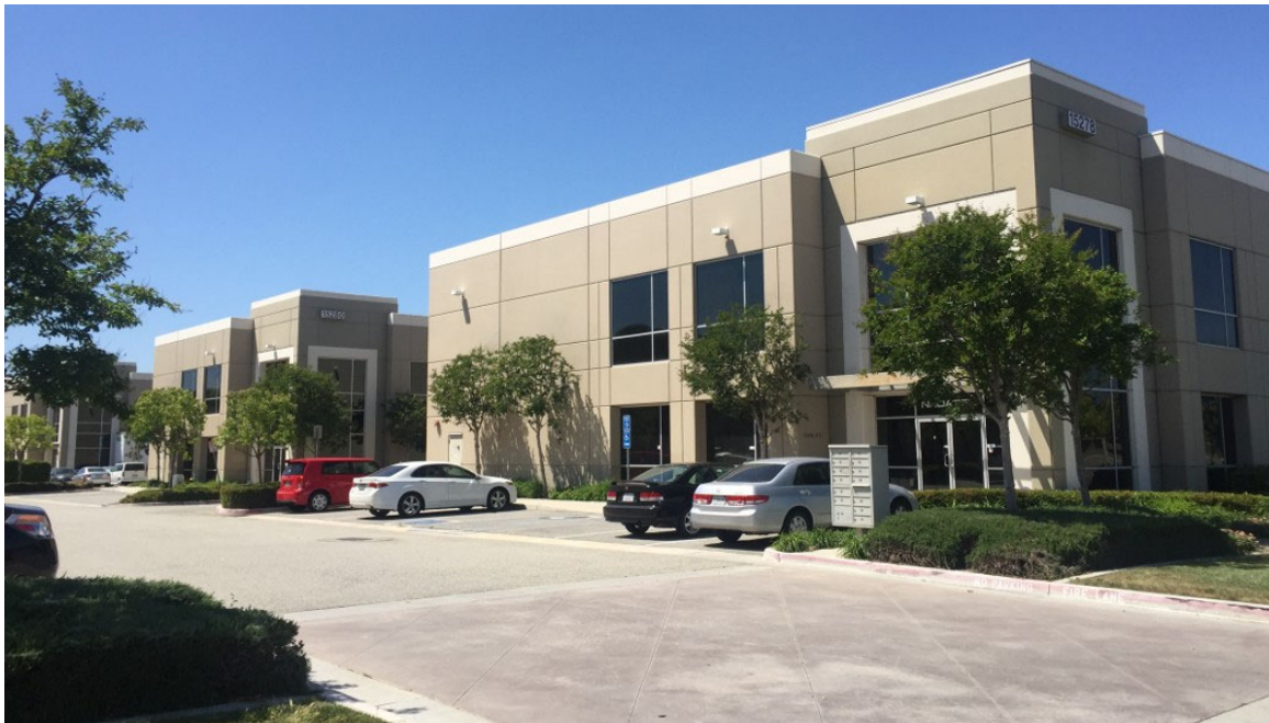
Photo 6.1 - Example of main building accents oriented towards street and entry
