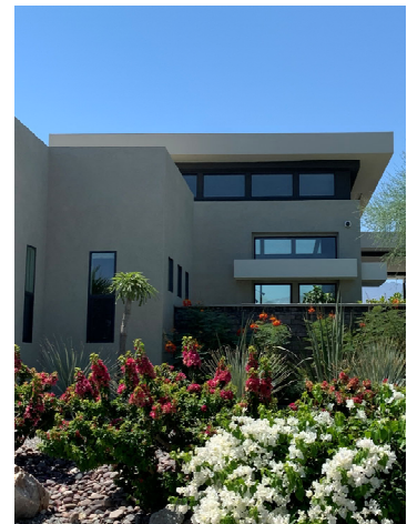
Horizontal windows under roof overhang and vertically oriented secondary windows.
