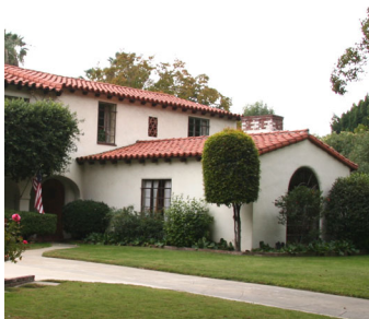
Contrasting dark brown fascia and window trim with pale stucco body and red "S" tile roof.
