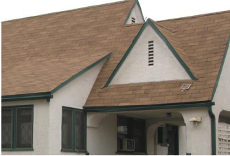
Steep roof pitches with articulated massing and gable end venting as accents.
