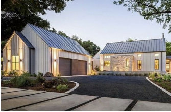
Simple roof forms with standing seam metal roof.
