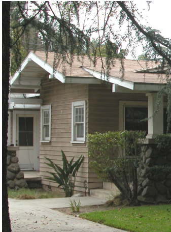
Low slope roof with large, exaggerated overhangs with wood supports and fascia.
