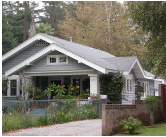
Low slope gabled roofs with large overhangs.
