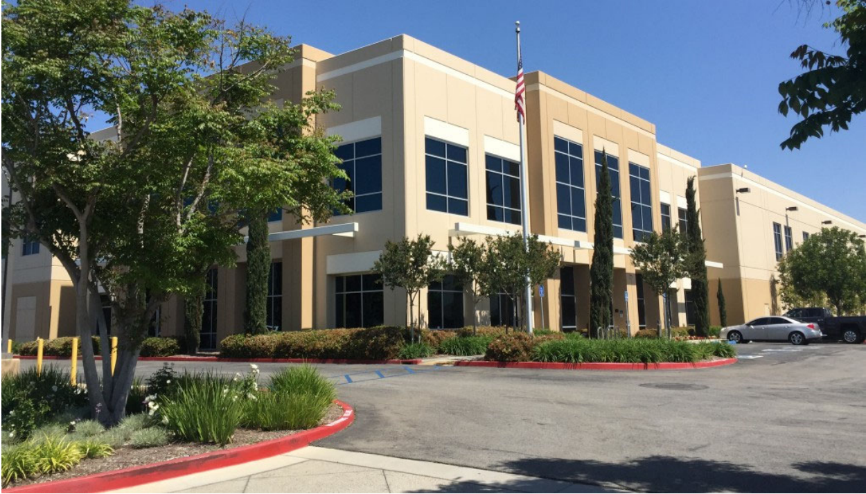
Photo 6.2 - Example of an Industrial edge along a perimeter street such as Hamner Avenue
