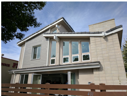
Concrete block vertical element and low pitched butterfly roof.
