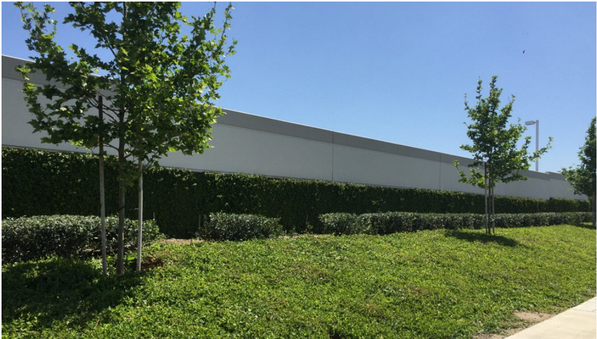
Photo 7.4-Example of typical screen wall with landscaping
