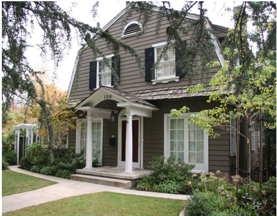
Barn shaped roof with coloring similar to siding is accented with bright white trim and dark shutters, use of large multi-paned French doors and windows.
