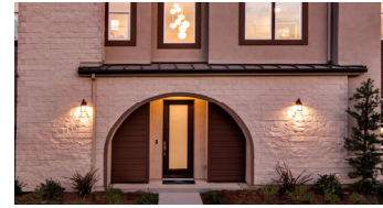
Entry porch with door on accent wall
