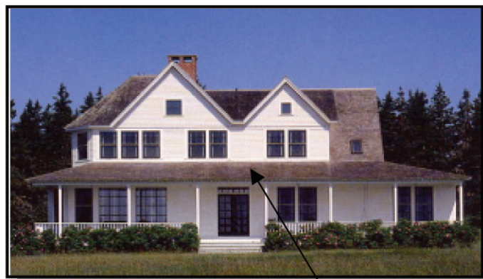
Porches along Front and Rear Elevations with a Shallow Roof Break
