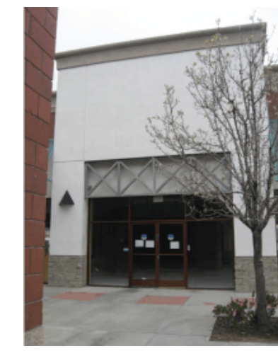
EXISTING CONDITION - SOUTH ELEVATION
