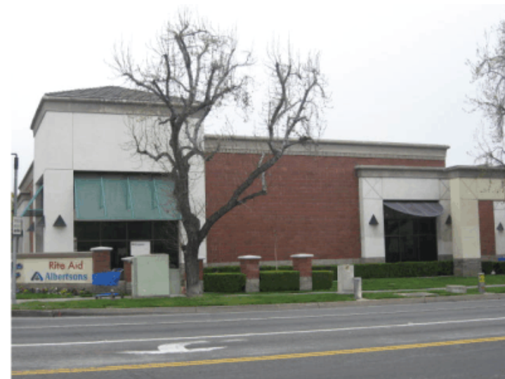
EXISTING CONDITION - WEST ELEVATION
