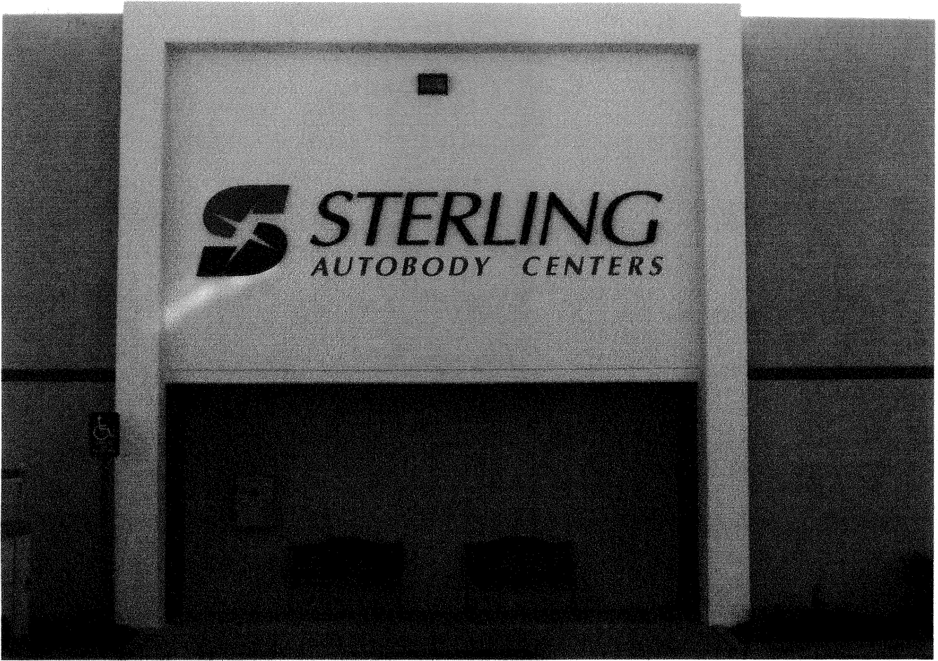
Example of Typical Sign Sterling Auto Body Building 4
