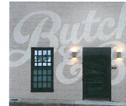
PAINTED LETTERS DIRECTLY ON TENANT STOREFRONT
