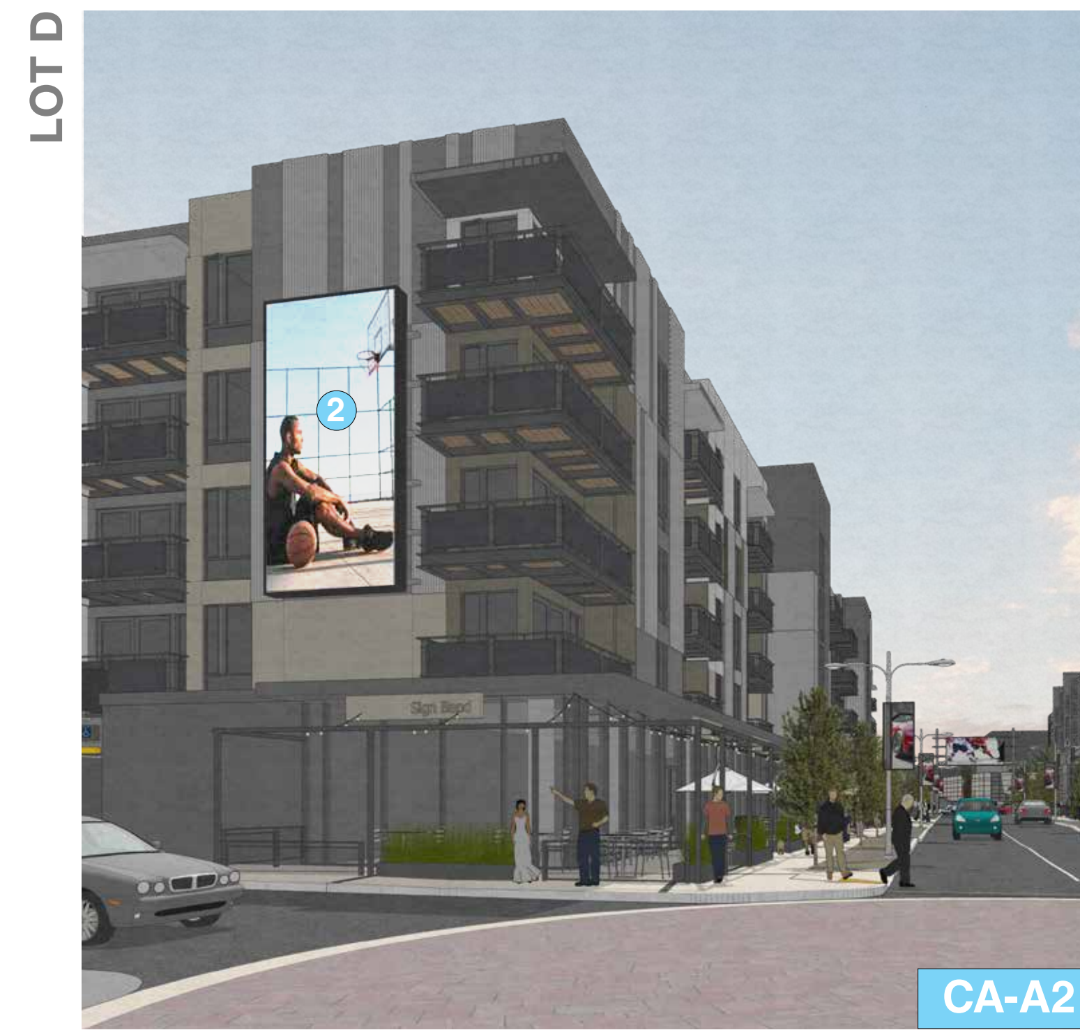
SIZE: 24' H X 12' W X 1'6" D HEIGHT OFF GROUND: 22'-0" AREA: 288 SF ATTACHMENT: WALL MOUNTED TO RESIDENTIAL STRUCTURE
