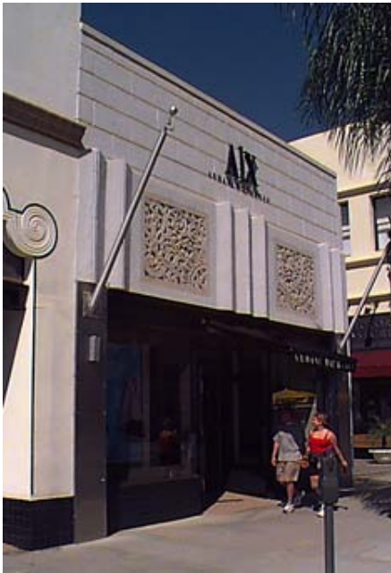
Vertical molding and facade detailing is typical of the Art Deco era.
