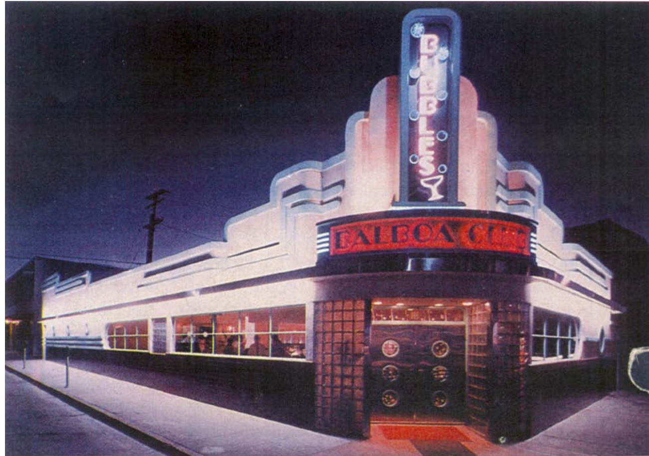
Example of a lit building from the 1920's - 40's time-period. Note the concealed lighting along the facade moldings, neon and internally lit signs.
