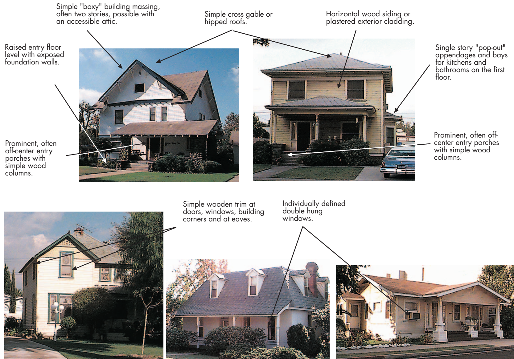
Figure 4.9: Wood-framed or Grove House – Style Characteristics
