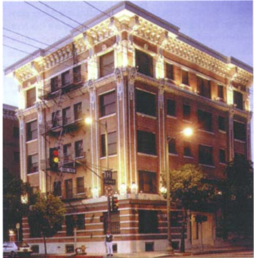
Example of a lit building from the turn-of-the-century period. Note the uplit cornice, the concealed lighting at the top of the pilasters, and the decorative fixture at the street level.
