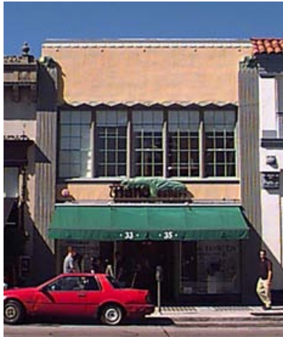
Vertical molding in the pilasters, horizontal molding at the parapet line and centralized facade are typical of this era.
