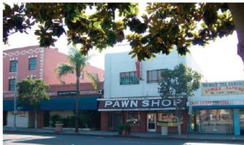
Lerch Building - Current photo showing front of building
