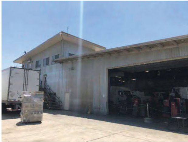
View of truck service building and office.
