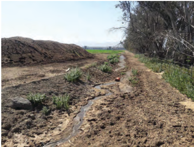
View of stormwater drainage swale.
