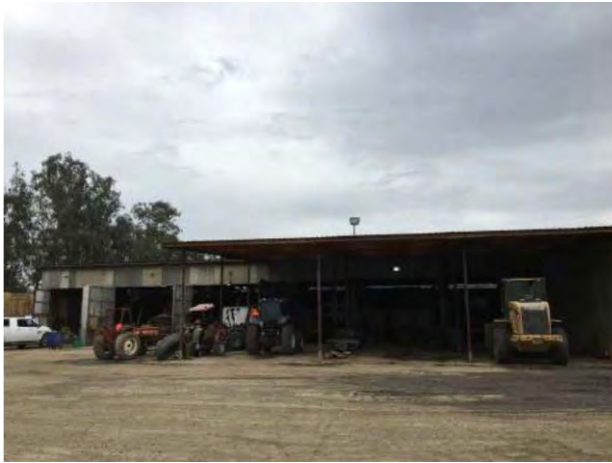
View of maintenance shop.
