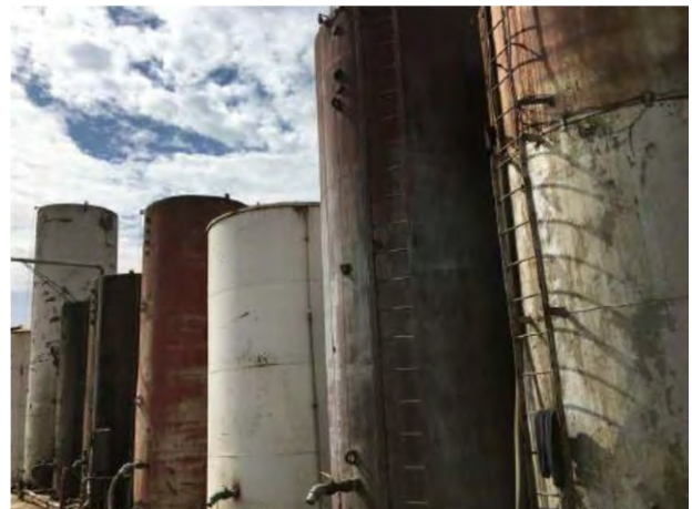
View of typical feed silos.
