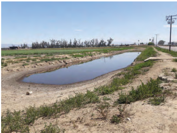
View of wastewater lagoon.
