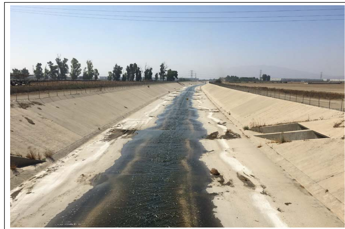
Photograph 8: View to the south of the Cucamonga Channel from the existing Merrill Avenue Bridge crossing.
