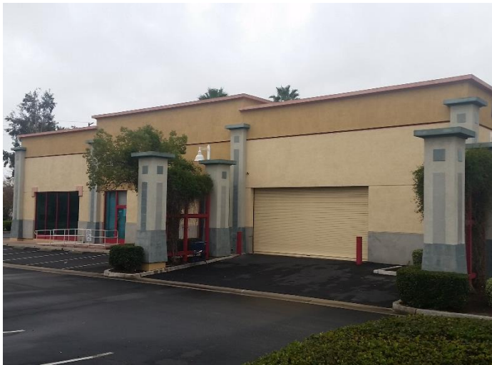
View of East Elevation (Proposed Patio Area)
