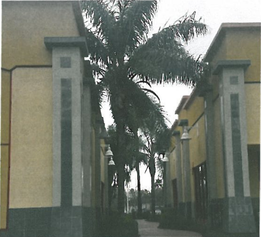
View of West Elevation (Paseo)
