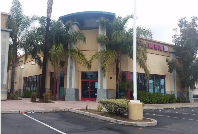
View of South Elevation (Entrance)
