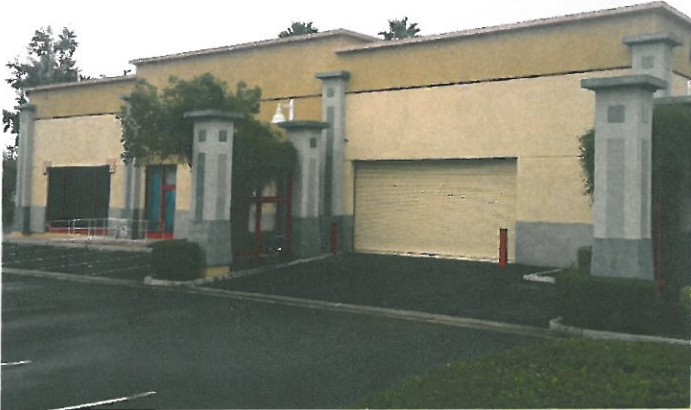
View of East Elevation (Proposed Patio Area)
