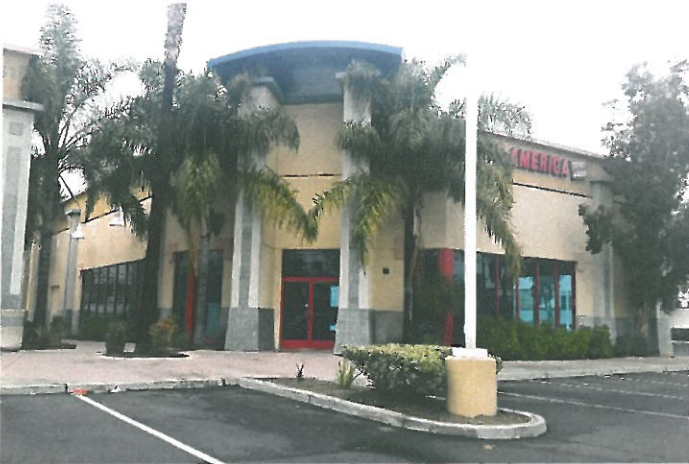
View of South Elevation (Entrance)
