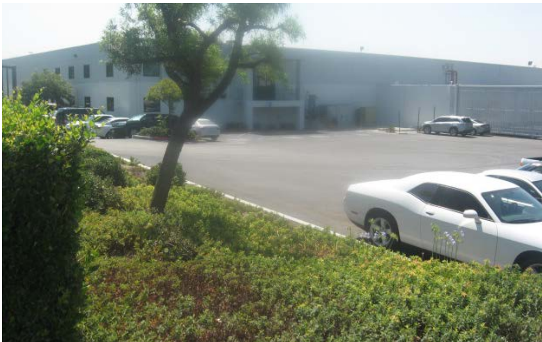
Southeast View of Adjacent Building at 5180 E. Airport Drive
