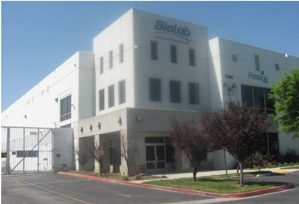
Southwest View of Building's Main Entrance
