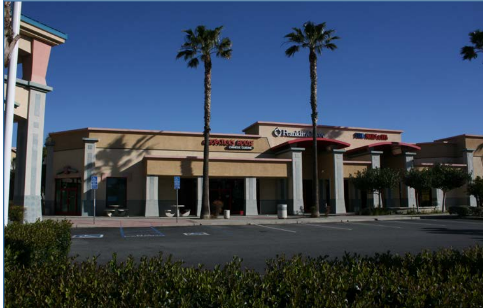
Above: South Parameter View of Project Site
