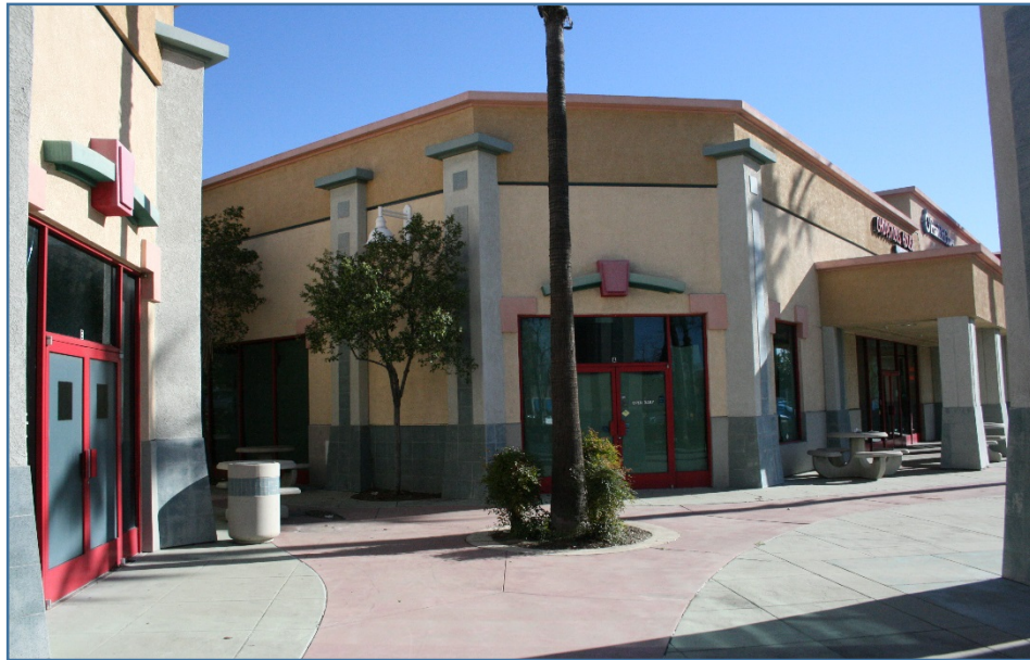
Above: View of South Elevation (Entrance)
