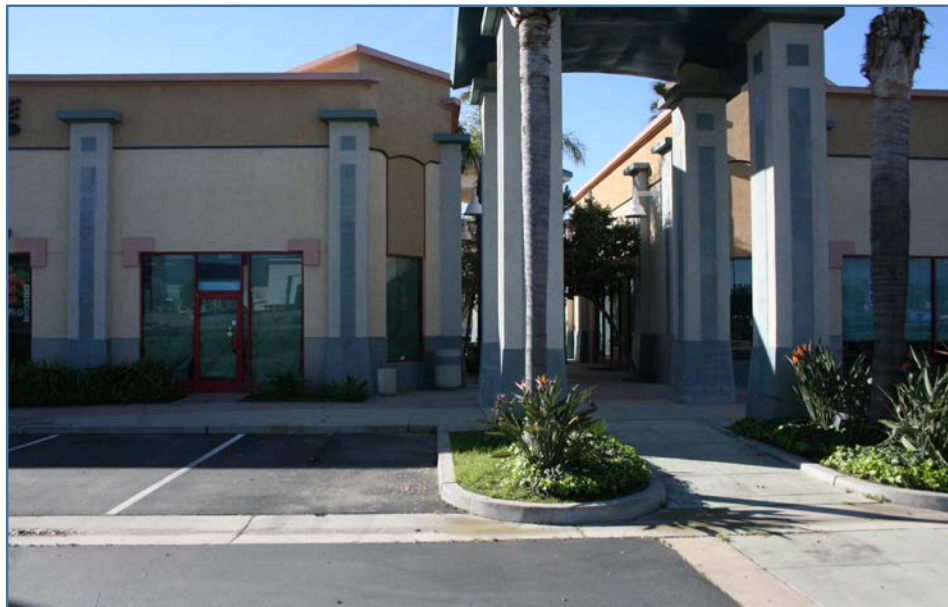
Above: View of North Elevation (Rear Entrance)
