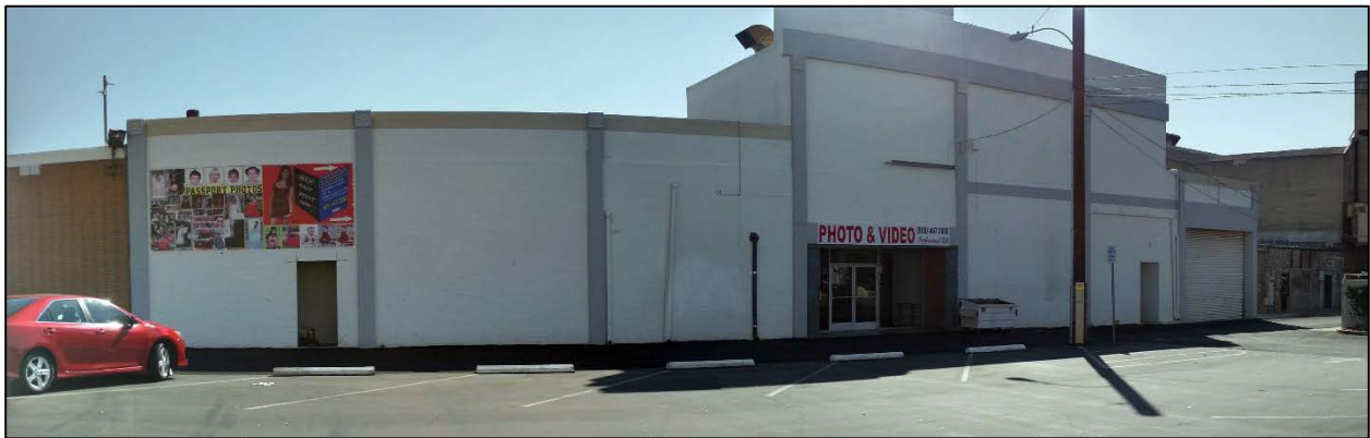
Project Site – Rear view looking east
