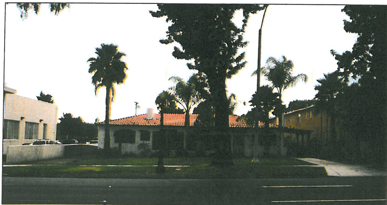
747 North Euclid Avenue (east elevation)
