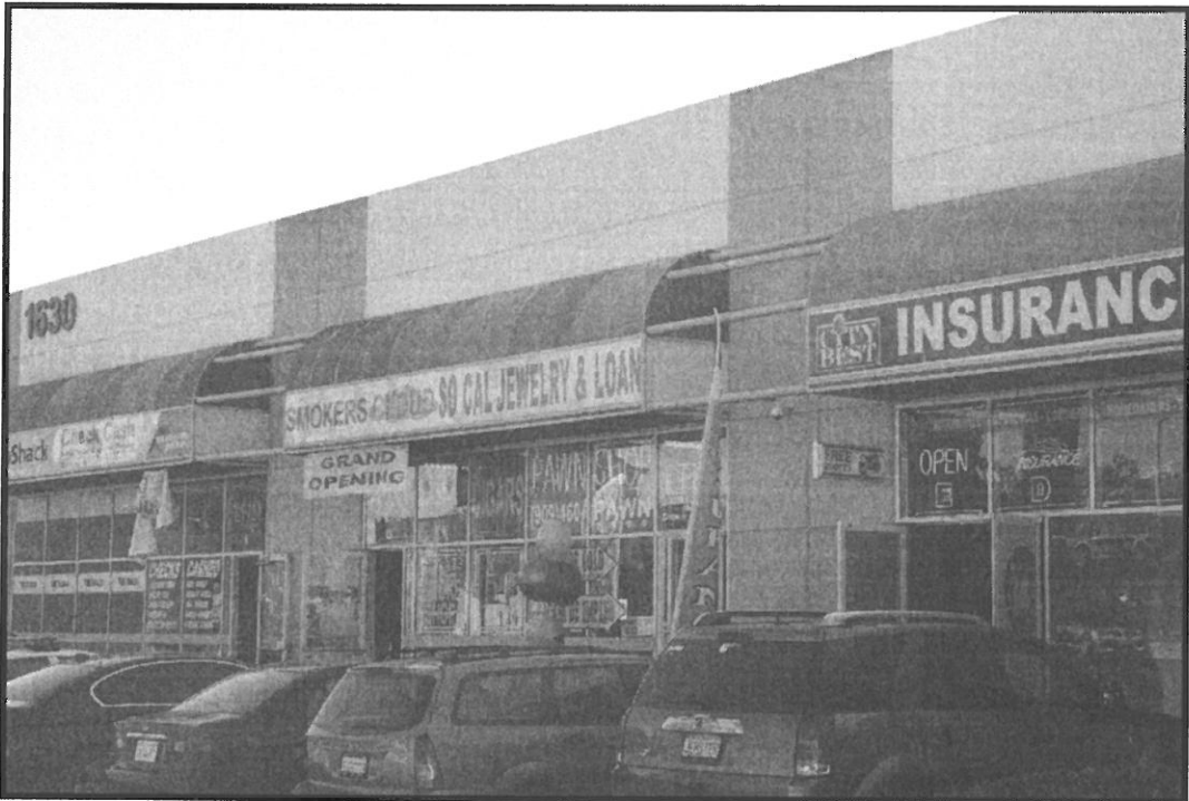
Existing Store Frontage (Tenant Space "F")
