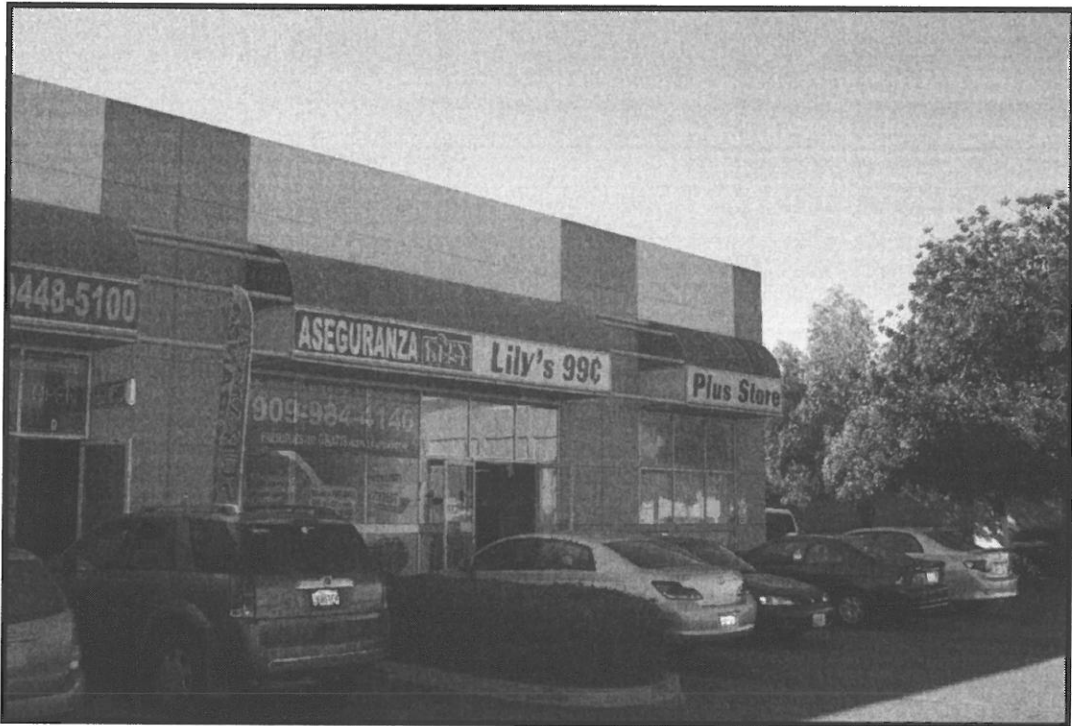
New Store Frontage (Tenant Space "AB")
