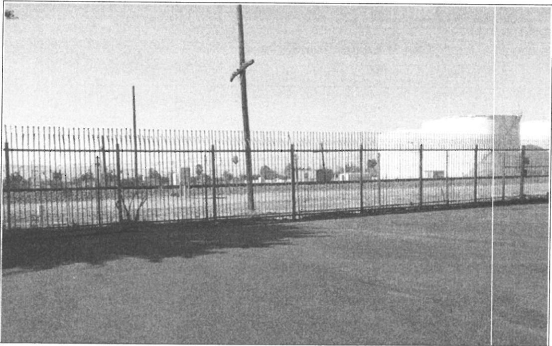
Rear Parking Lot-Looking South
