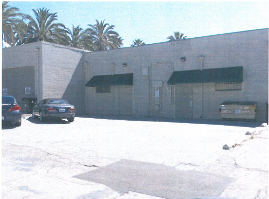
View of Rear of Subject Building and its Parking Lot
