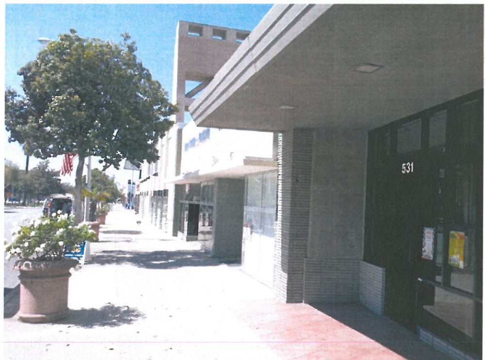
View of Front of Building Looking South on Euclid Avenue
