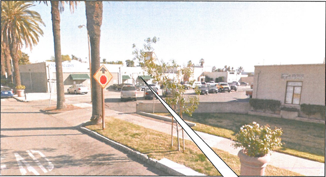
View of Rear of Building and Parking Lot Areas
