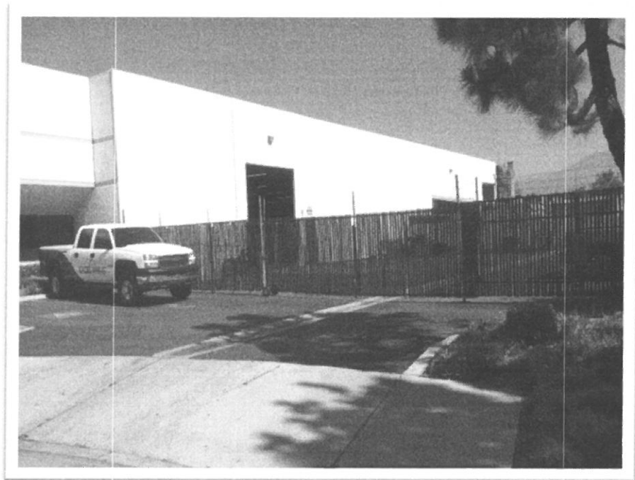
View of Existing Chain link Fence
