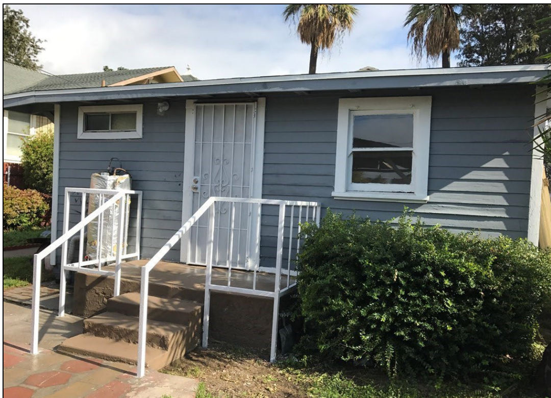
Rear – View looking northeast
