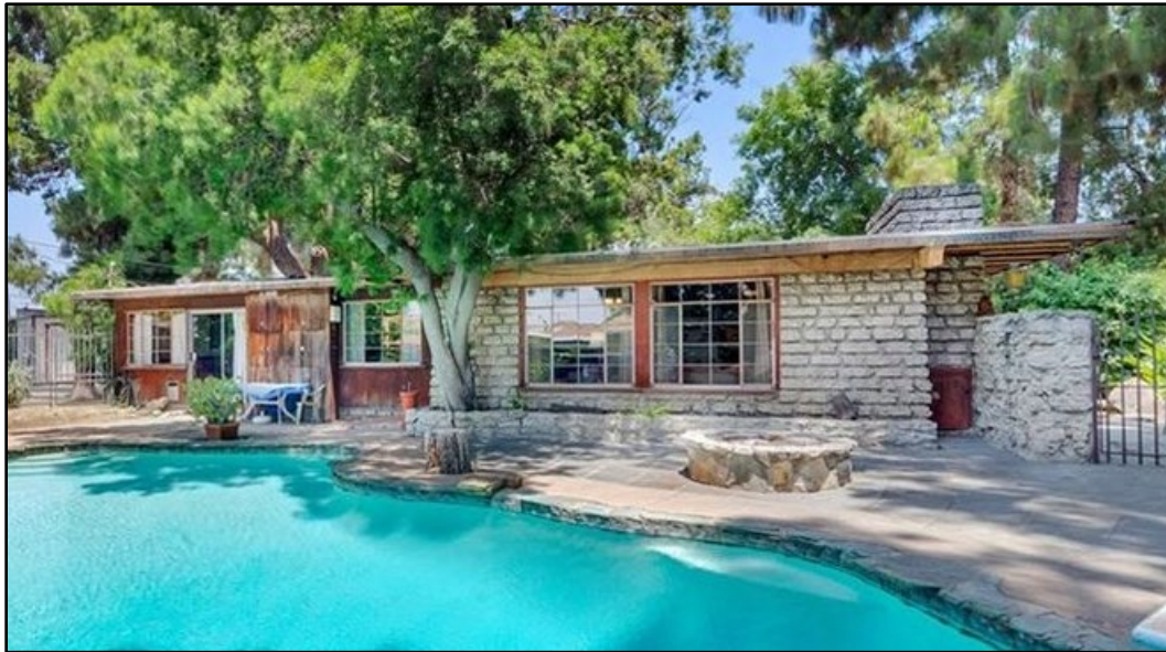
Figure 3: Maurice Johnson House Rear, view looking east
