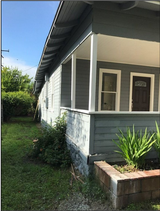
South façade, view looking northwest
