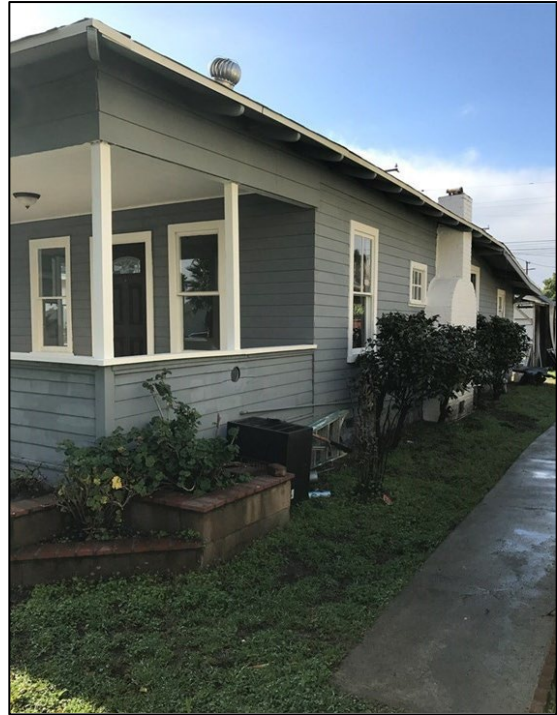
North façade, view looking southwest
