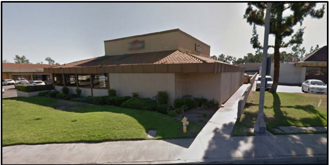
Northeast corner of Existing Building
