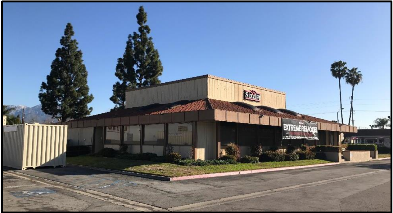
Southwest corner of Existing Building
