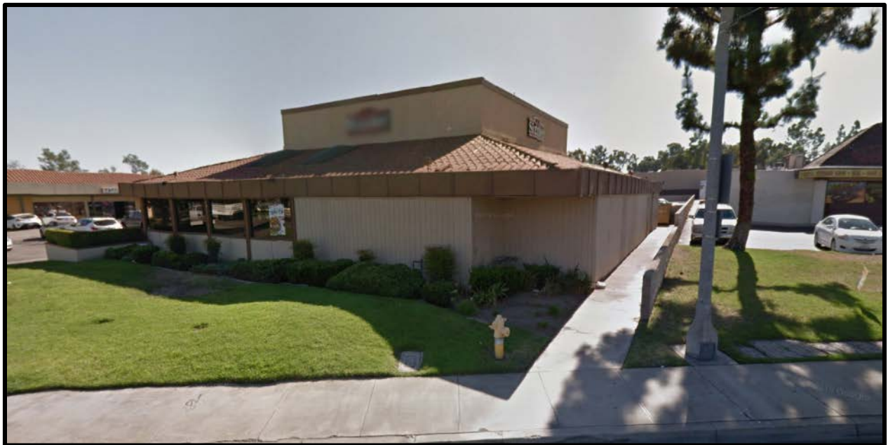
Northeast corner of Existing Building
