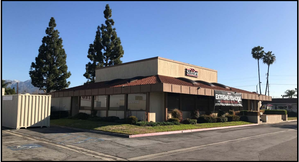
Southwest corner of Existing Building
