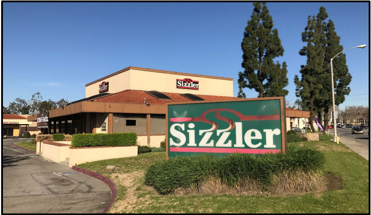
Southeast corner of existing building
