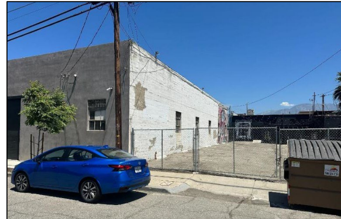
East elevation view looking northwest
