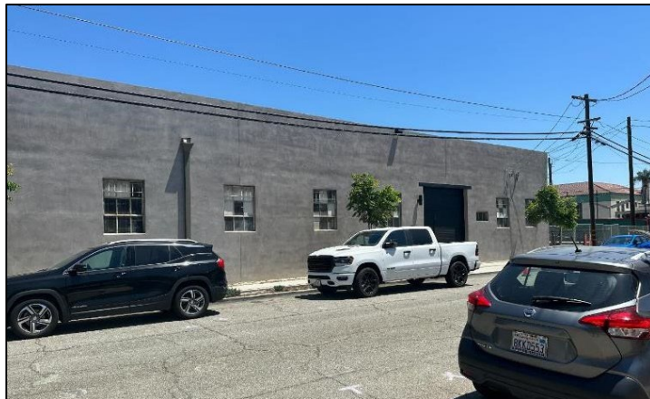
South elevation view looking northeast
