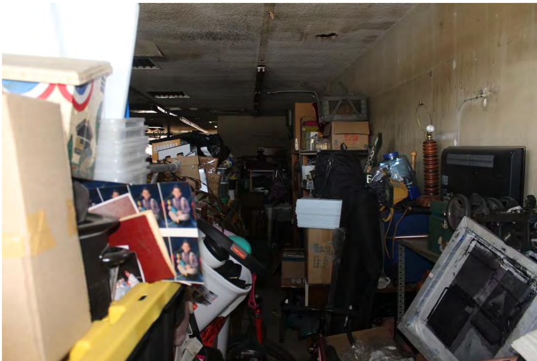
Overview of inside former dry cleaner unit.
