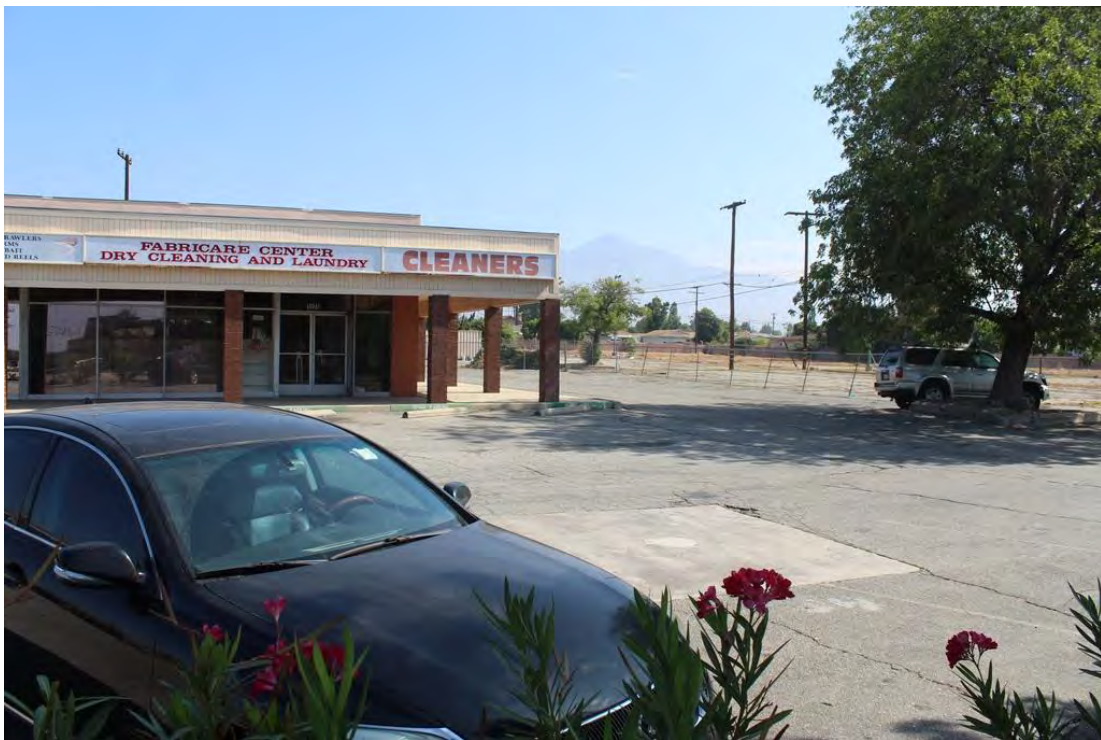
Overview of Ontario Plaza Mall looking northeast.
