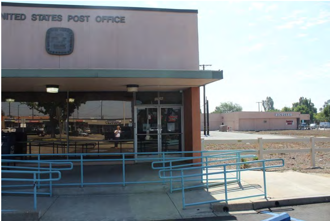
Overview of post office looking east.
