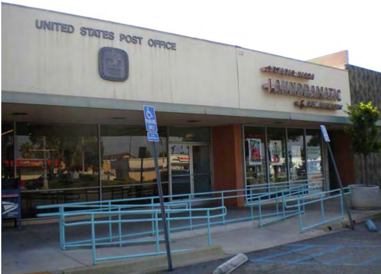
Figure 2: Photograph of the Plaza Center Station and the part of Ontario Plaza that was demolished in 2014, 2009 (David Allen).
