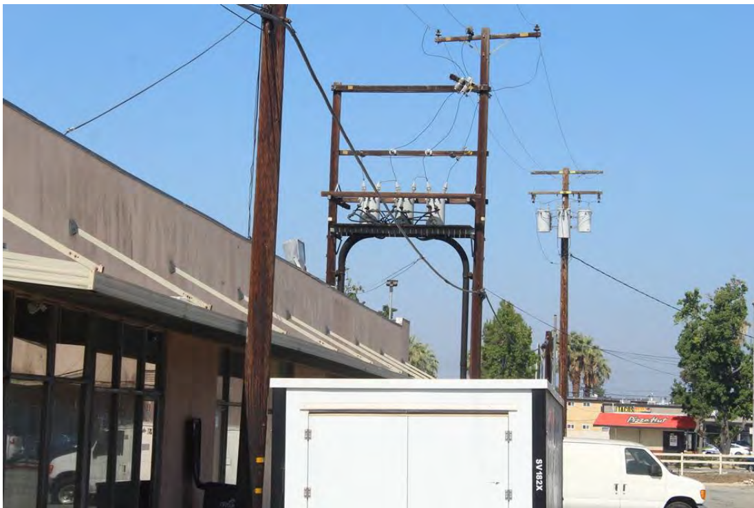
Overview of site looking west with power poles
