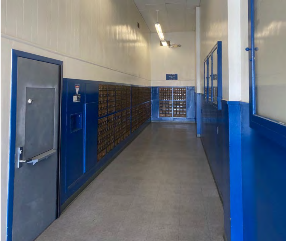
Photograph 5: 1126 N Mountain Ave post office interior hallway, April 24, 2023.
