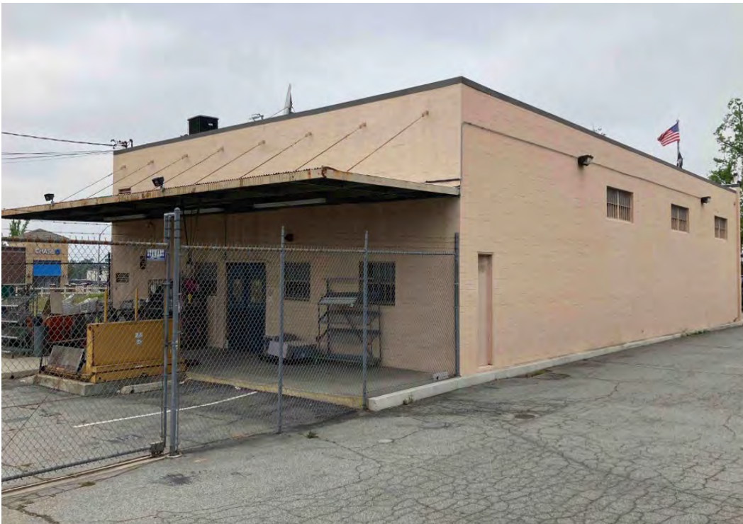
Photograph 3: 1126 N Mountain Ave, east and north elevations, camera facing southwest, April 24, 2023.
