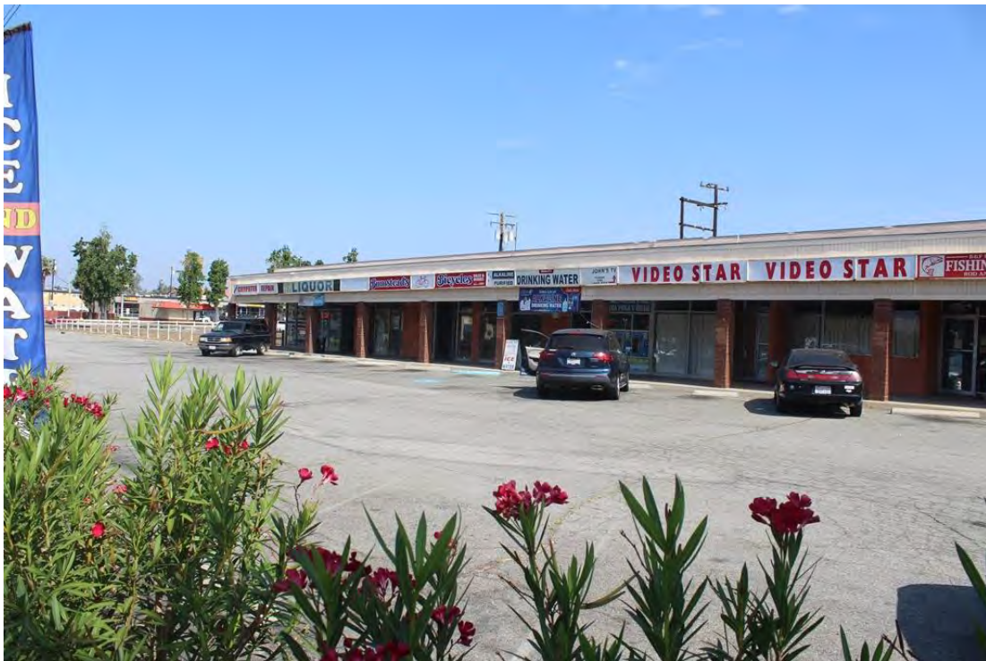
Overview of Ontario Plaza Mall looking northwest.
