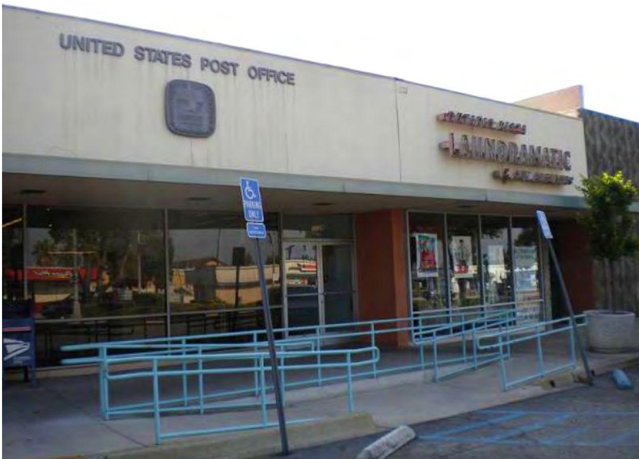
Figure 2: Plaza Center Station and the section of Ontario Plaza that was demolished in 2014, 2009 (David Allen).
