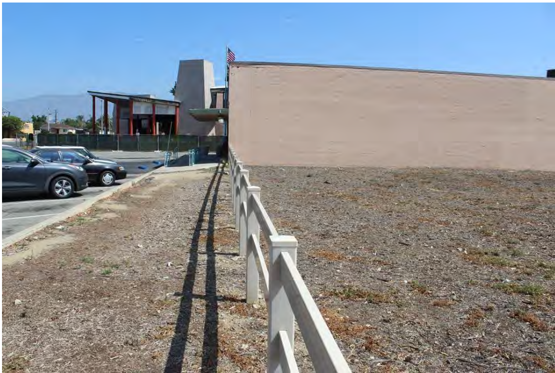
Overview of post office looking north.
