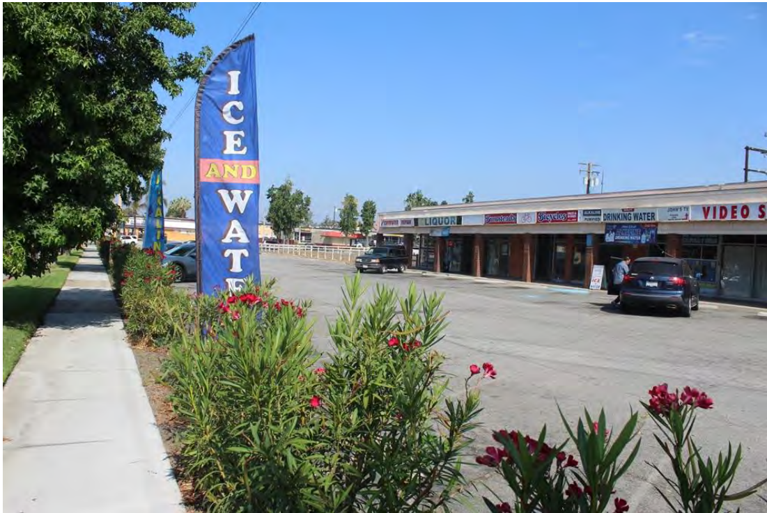
Overview of Ontario Plaza Mall looking northwest.
