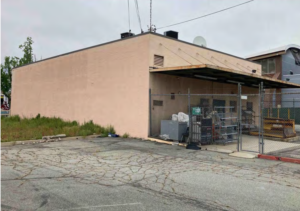
Photograph 2: 1126 N Mountain Ave, south and east elevations, camera facing northwest, April 24, 2023.
