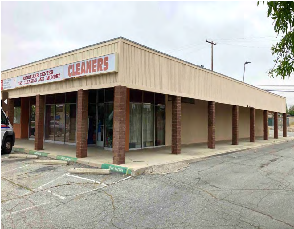
Photograph 4: Ontario Plaza Shopping Center, south and east elevations, camera facing northwest, April 24, 2023.
