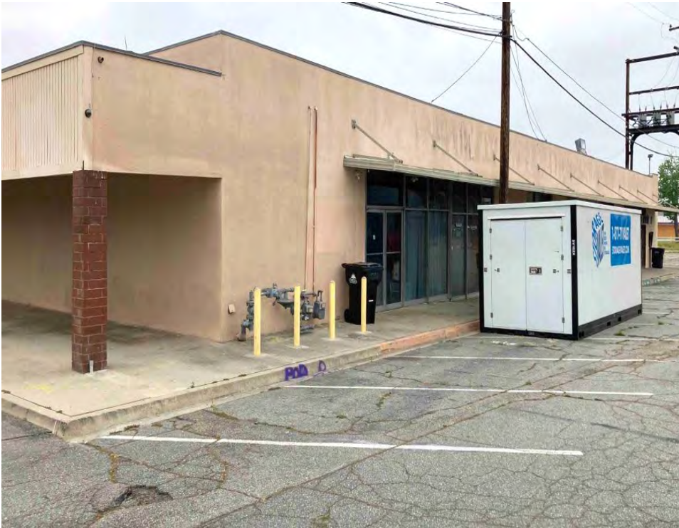
Photograph 5: Ontario Plaza Shopping Center, north elevation, camera facing southwest, April 24, 2023.
