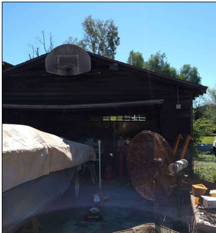
Existing Detached Garage
