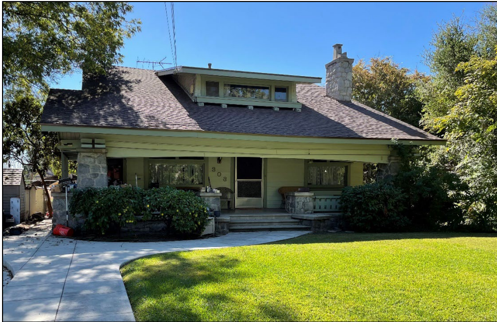
Charlotte Reed House - View looking southwest
