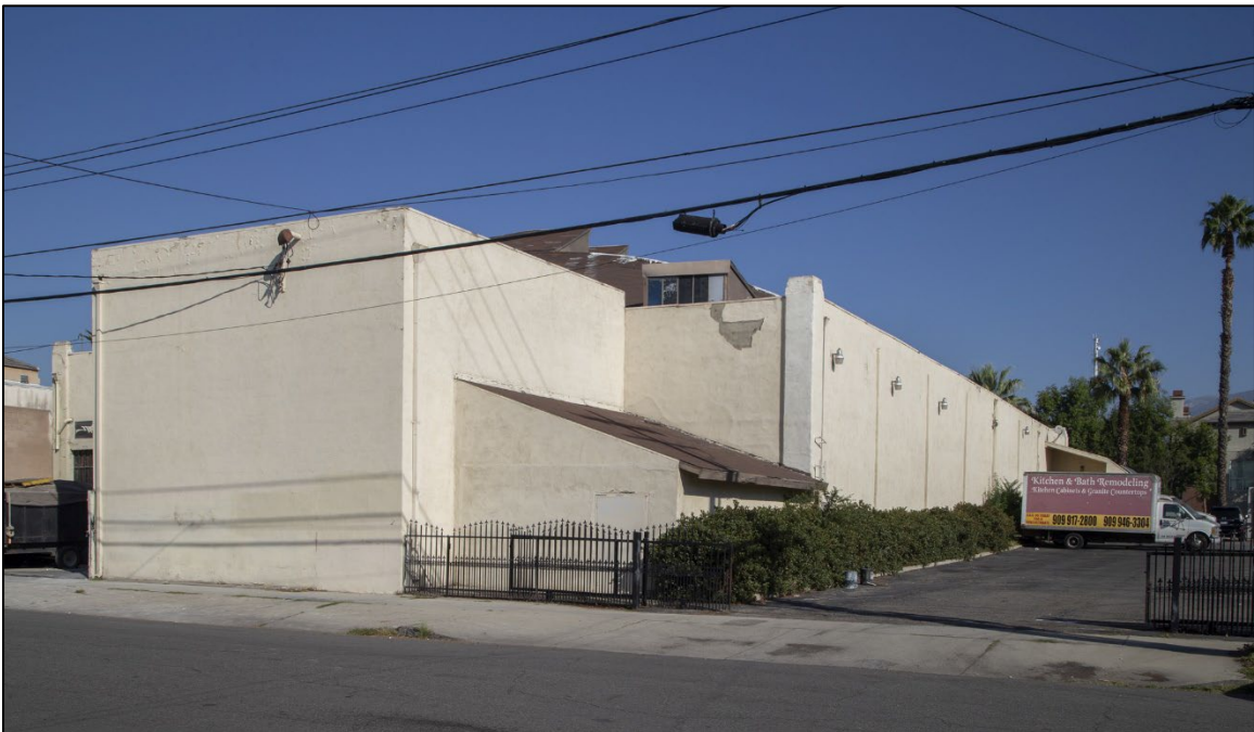
444 East Holt Blvd. – View looking northwest
