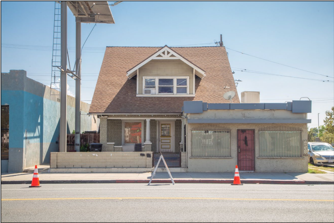
616-618 East Holt Blvd. – View looking northwest
