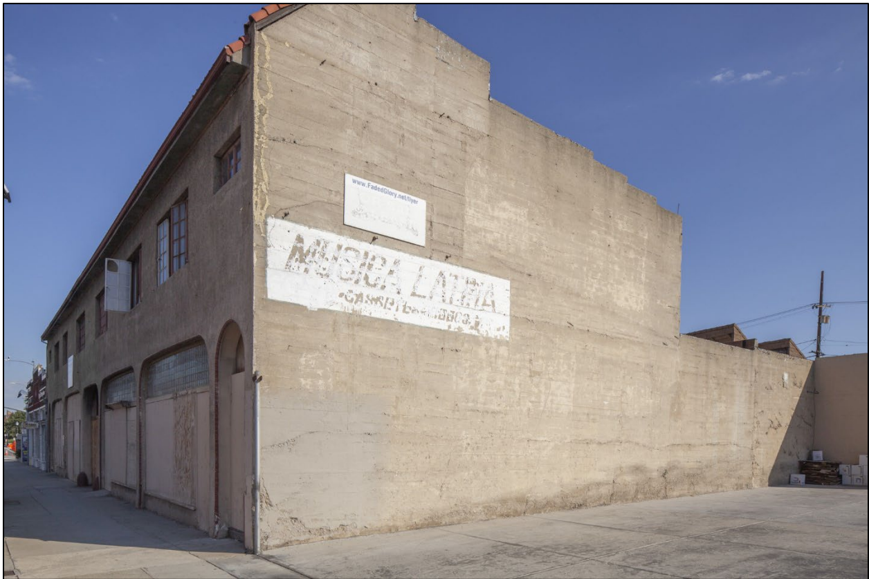
212-214 East Holt Blvd. – View looking southeast
