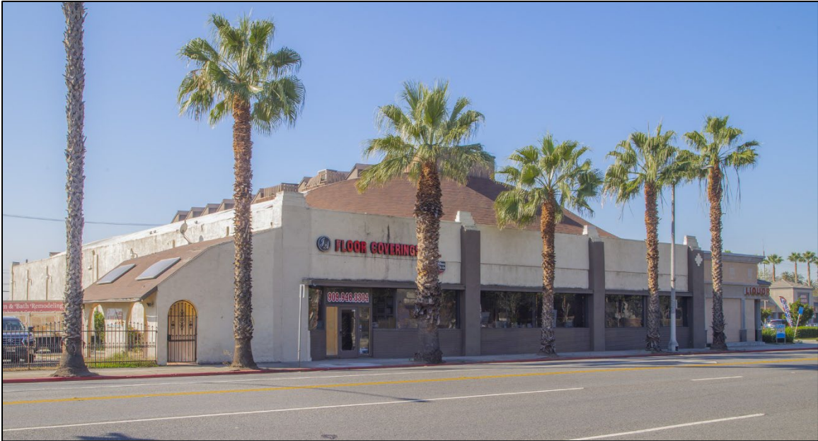
444 East Holt Blvd. – View looking southwest
