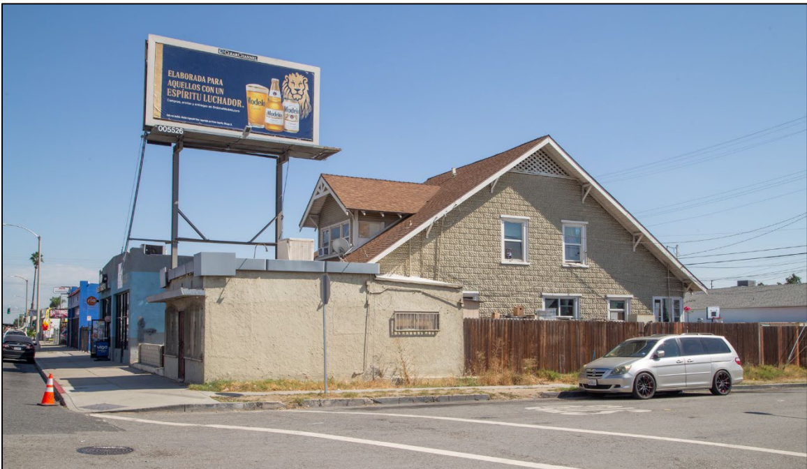
616-618 East Holt Blvd. – View looking southeast
