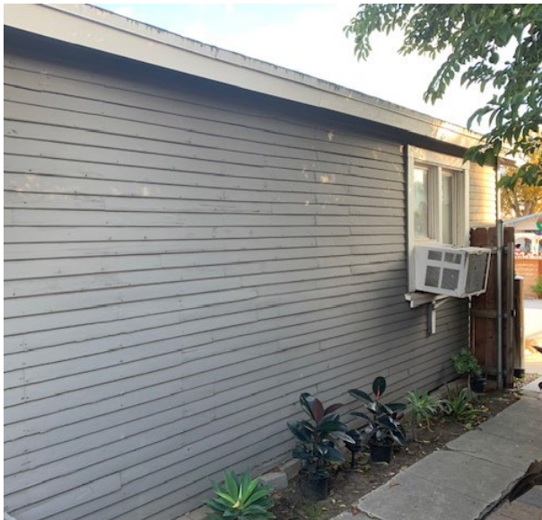
West façade, view looking southeast
