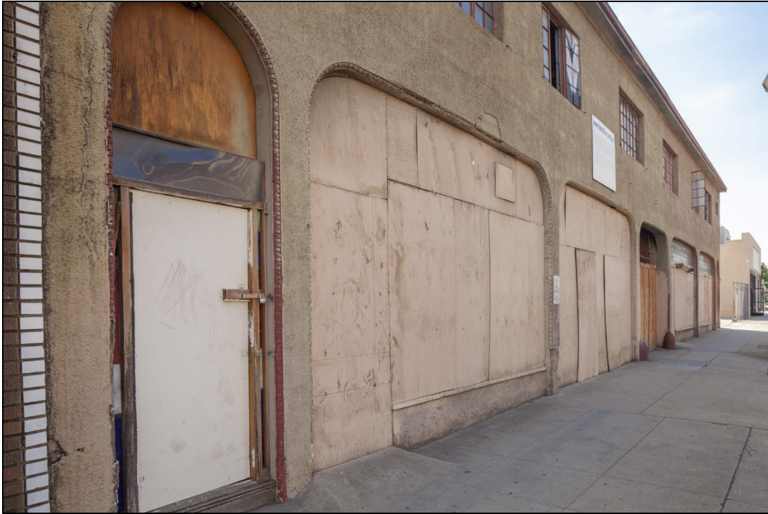
212-214 East Holt Blvd. – View looking southwest
