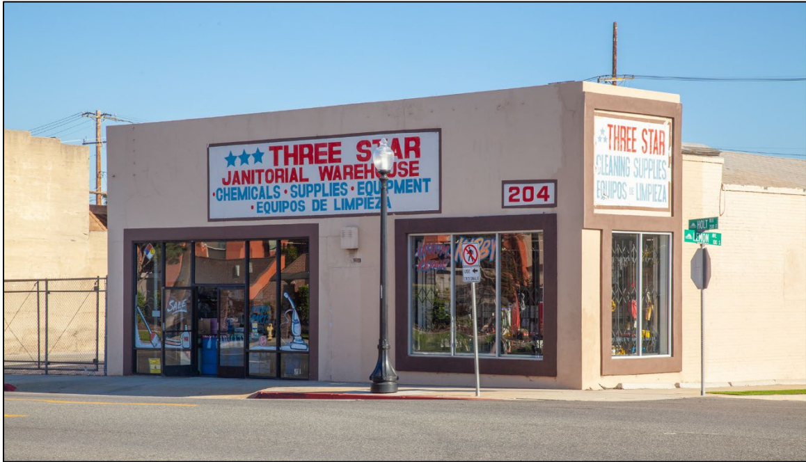
204 East Holt Blvd. – View looking southeast
