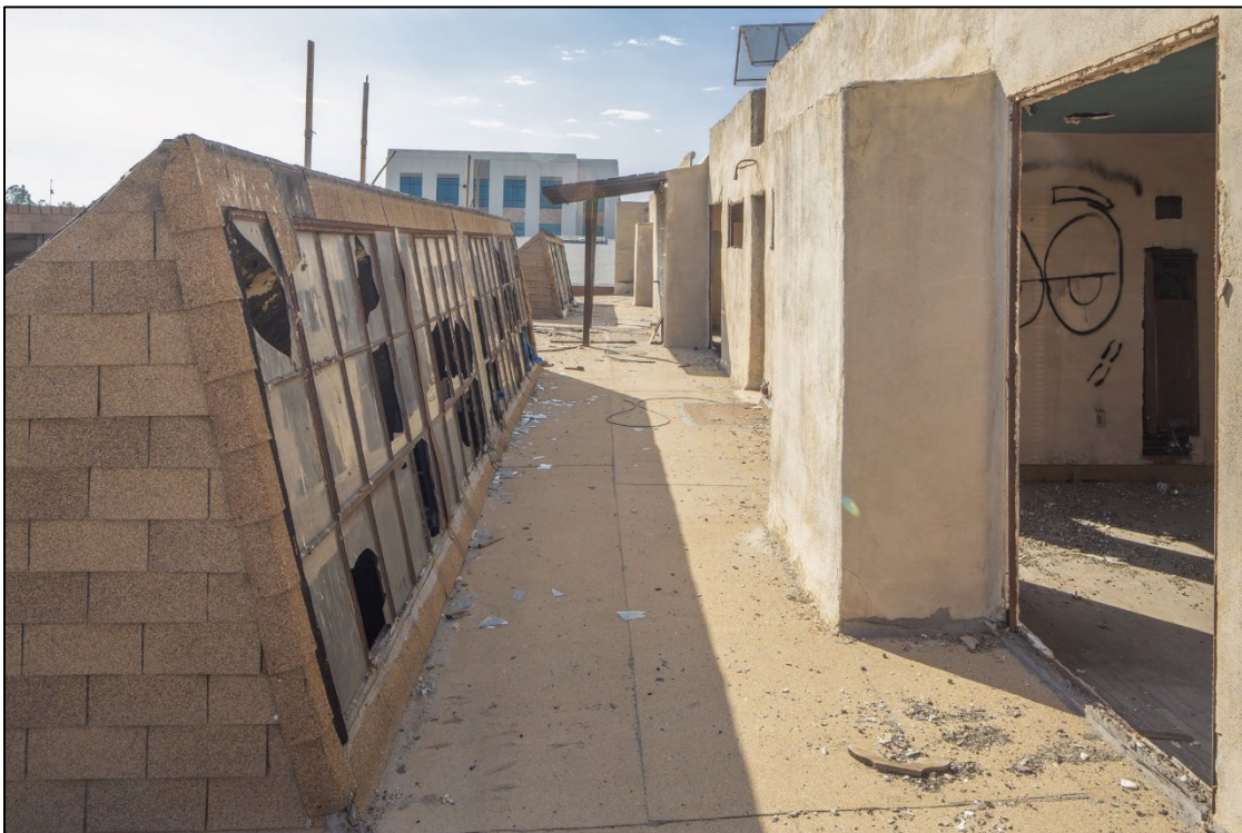
212-214 East Holt Blvd. – Roof, view looking west
