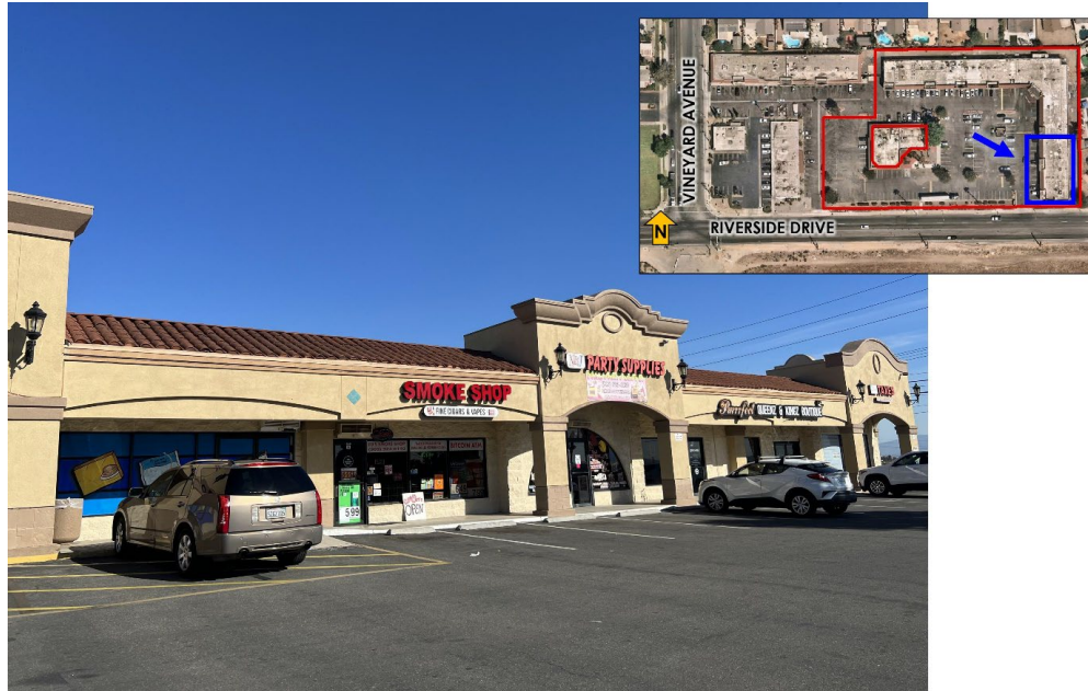
Existing shopping center Units 16-20 facing southeast.
