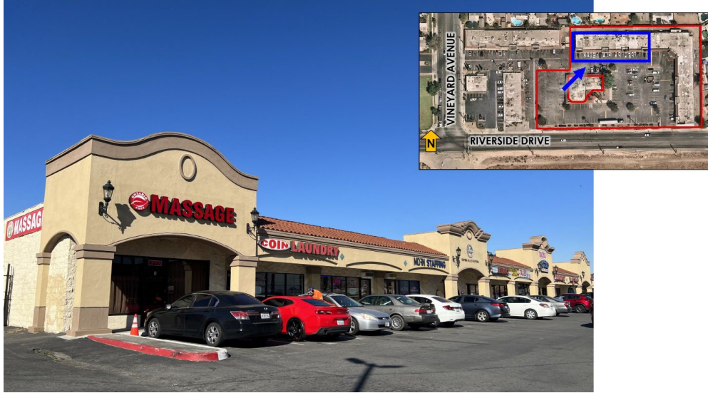
Existing shopping center Units 1-7 facing northeast.
