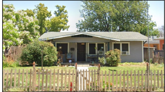
Figure 17: 638 North Allyn Avenue
