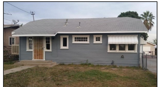
Figure 7: 602 North Allyn Avenue
