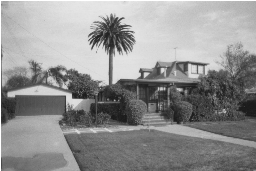
1984 Historic Resource Survey (view looking southeast)
