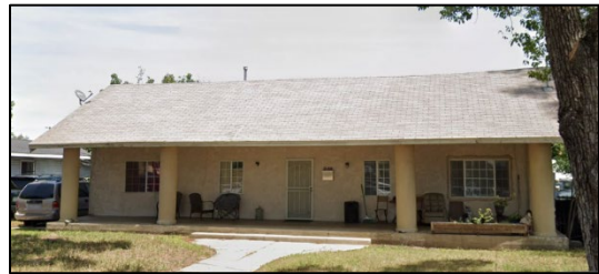
Figure 3: 500 North Allyn Avenue
