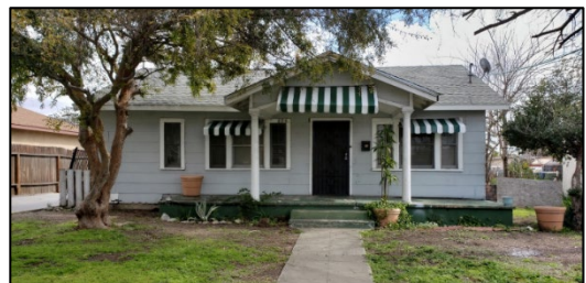
Figure 15: 624 North Allyn Avenue
