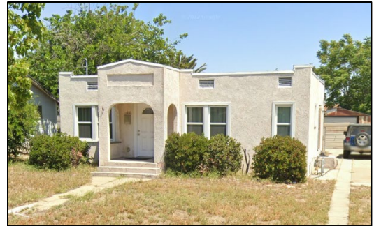
Figure 9: 618 North Allyn Avenue
