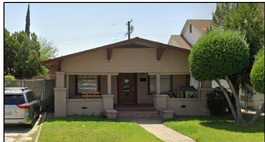
Figure 9: 906 East D Street
