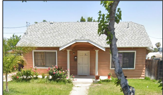
Figure 5: 614 North Allyn Avenue
