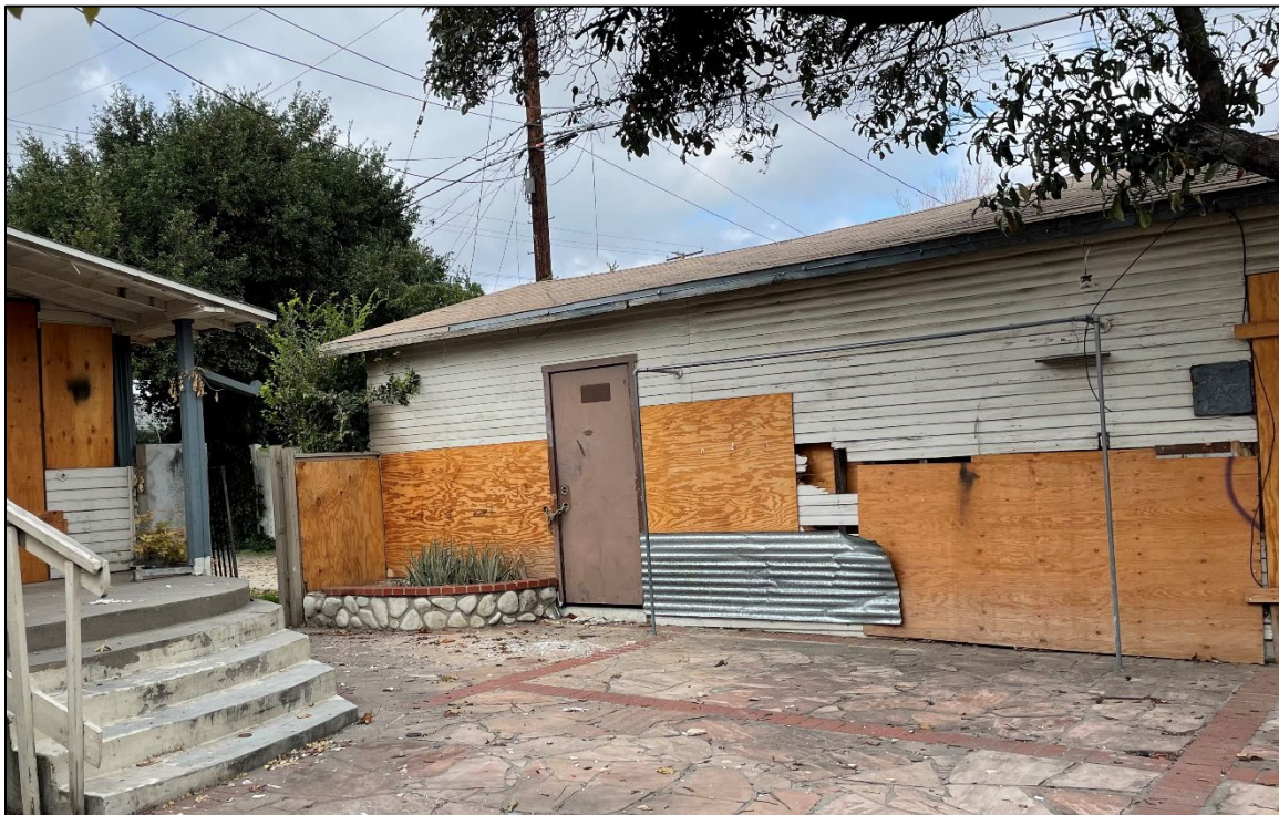
Garage – view looking north
