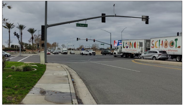
28 Photo looking west from the cross section of S Haven Avenue and E Airport Drive.
