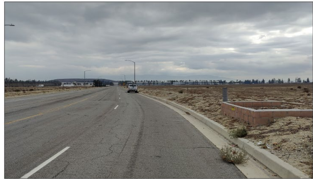
3 Photo looking south along S Carnegie Ave between E Airport Drive and E Santa Ana Street.
