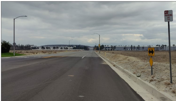
7 Photo looking south from S Carnegie Ave near Santa Ana Street.
