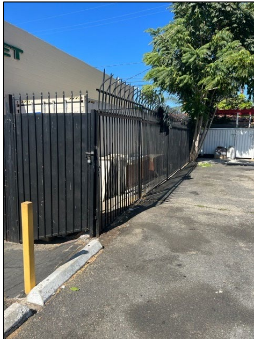
NORTH PROPERTY LINE, LOOKING WEST
