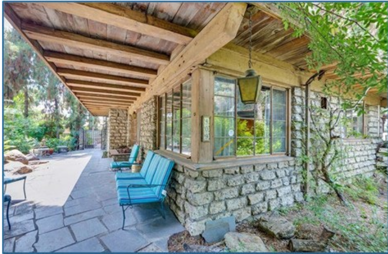
Image 1: View looking west Primary entrance
