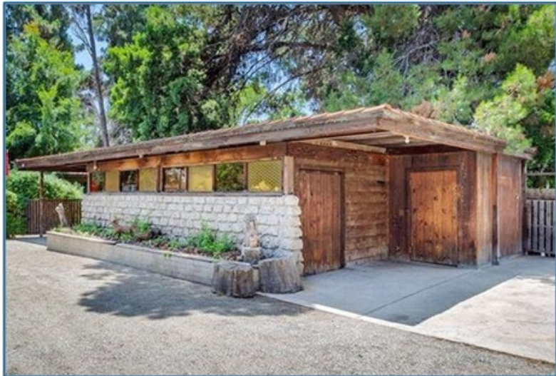
Image 3: Detached Garage, east elevation
