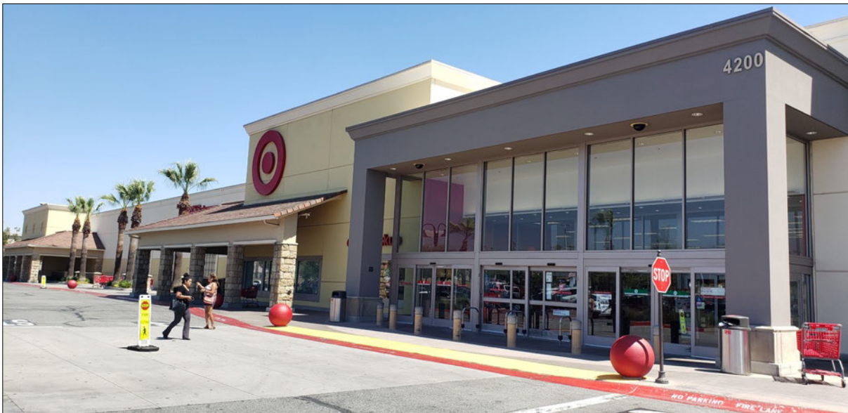
Target store entrance along northern portion of the building.
