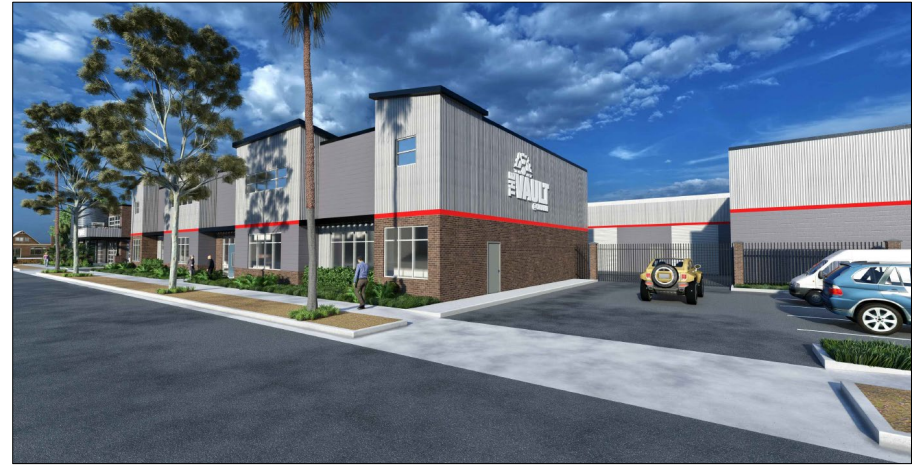
Northeast Corner of the Project Site
