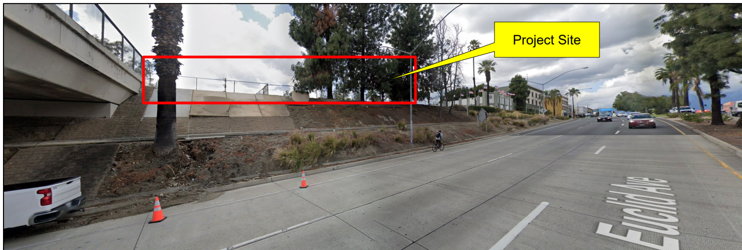
Euclid Avenue facing Northwest
