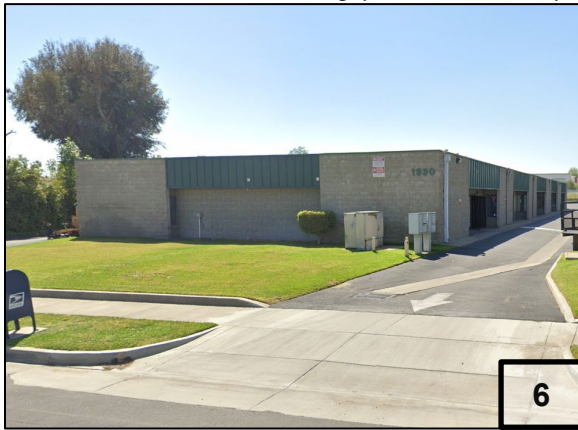
South Multi-Tenant Building Built 1986
