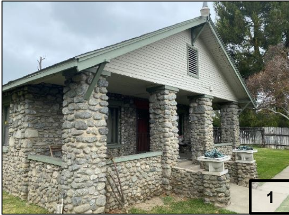
Primary Façade – East Elevation
