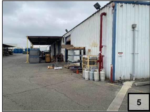
Northern Industrial Building (Built 1966-1980)
