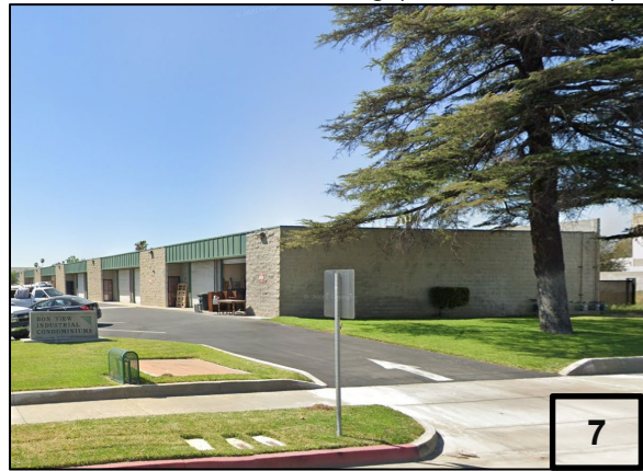
North Multi-Tenant Building Built 1986
