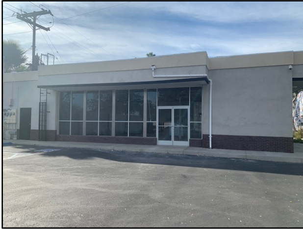
Figure 1: Street View of Project Site
