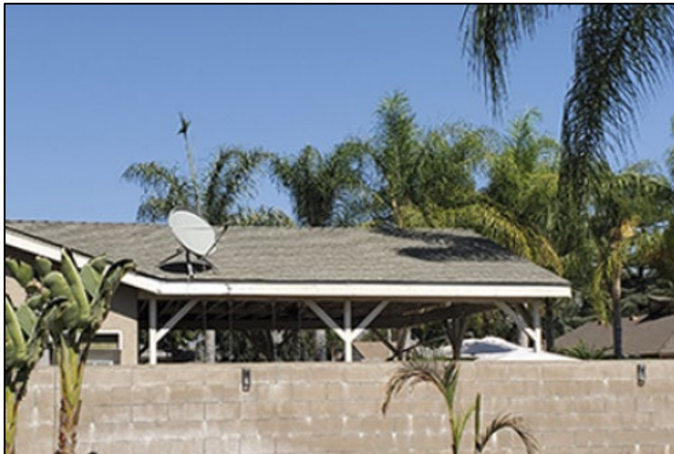
Looking North at patio cover from adjoining property.
