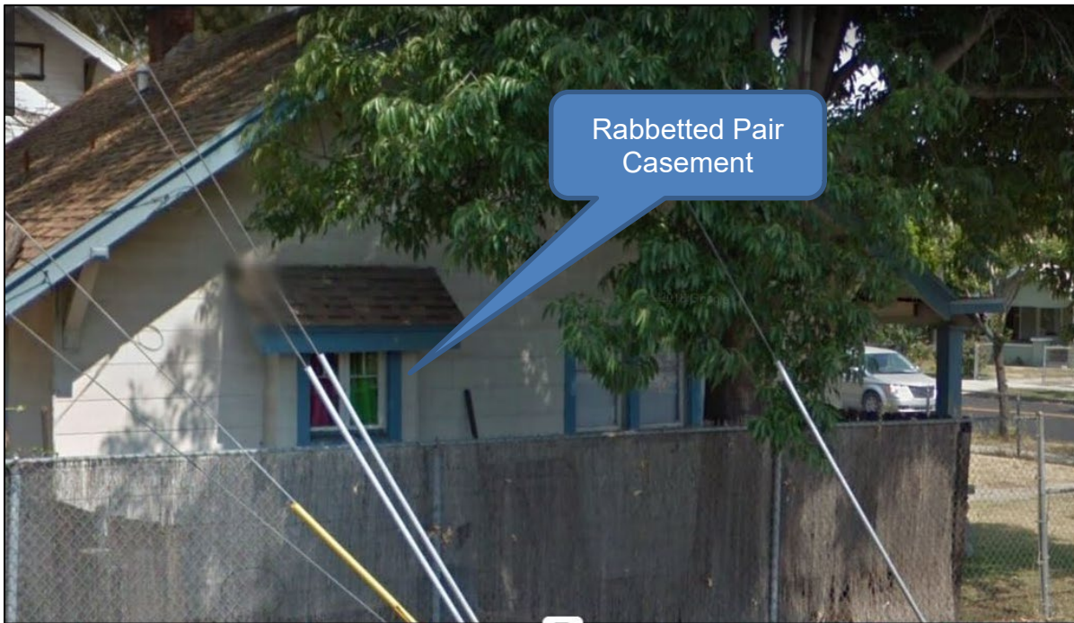
West Elevation (2006)- Window No. 5 (Bedroom)
