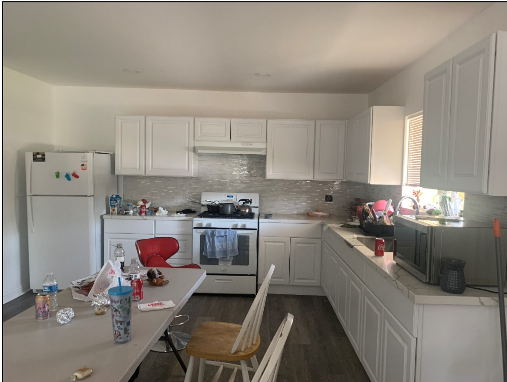
Kitchen Looking East- Window No. 1 (Removed)
