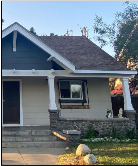
South Elevation- Window No.2
