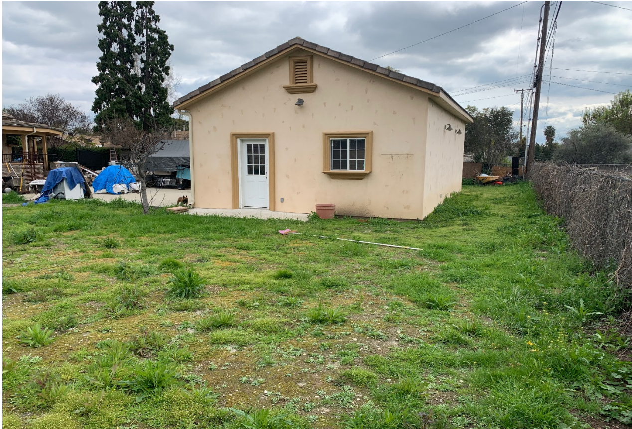
North View of the Existing 3-Car Garage
