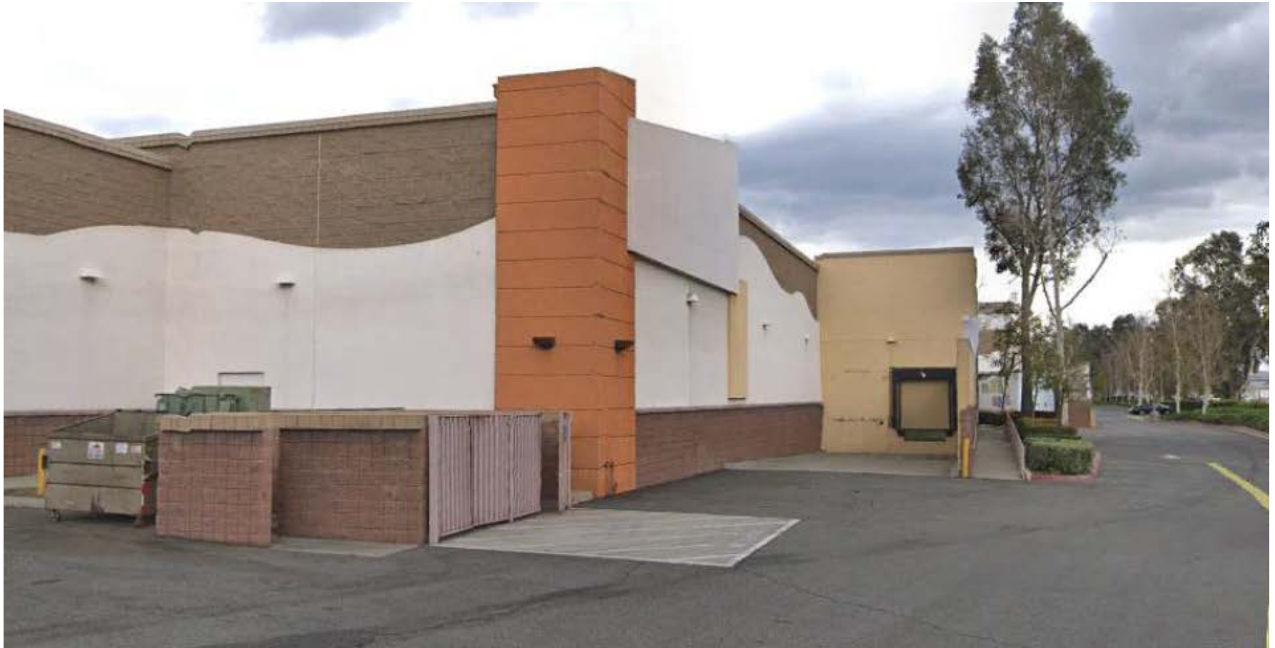
West View of the Existing Loading Dock Area
