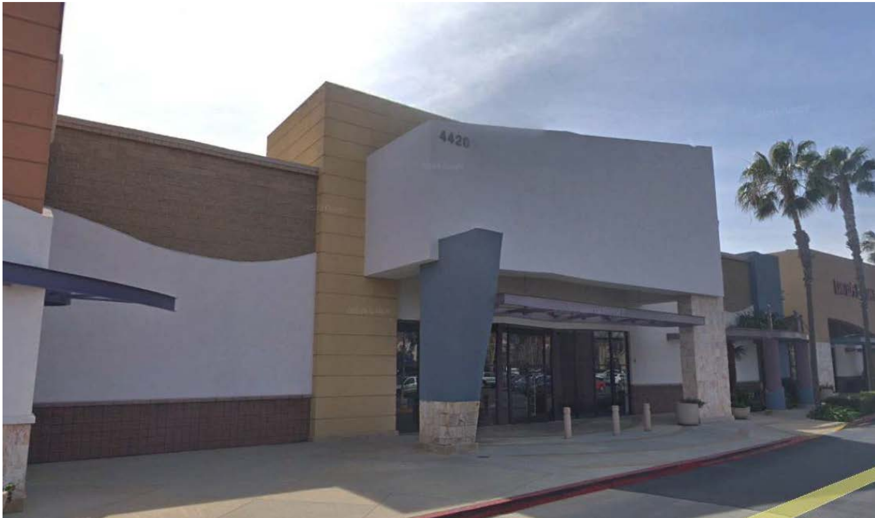
Grocery Outlet's Main Entrance (North Elevation)
