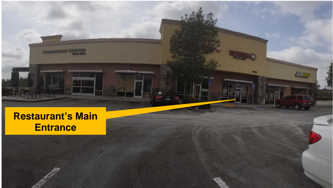
Northwest View of the Multi-Tenant Building
