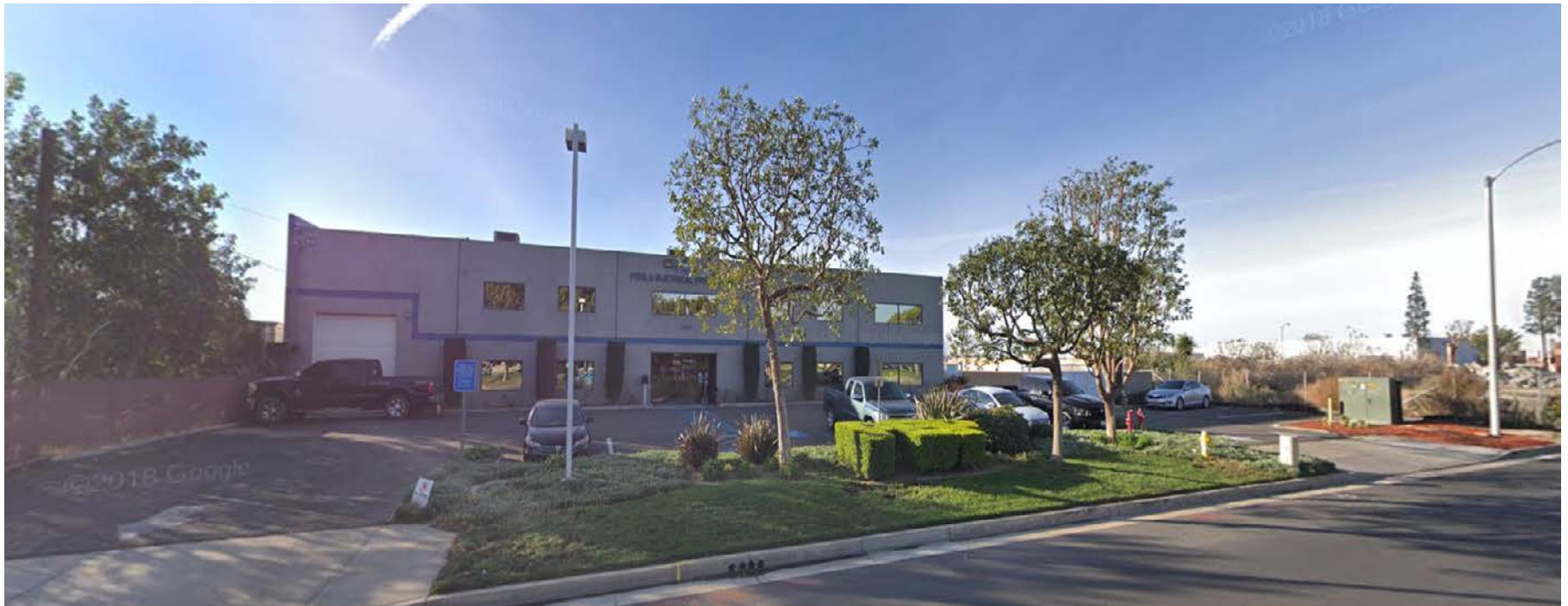
Existing Industrial Building – Looking Southwest from the Project Site
