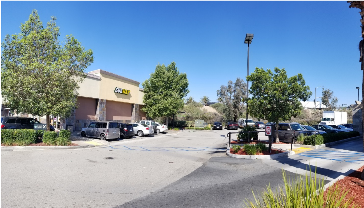
North View of Building & Parking Area
