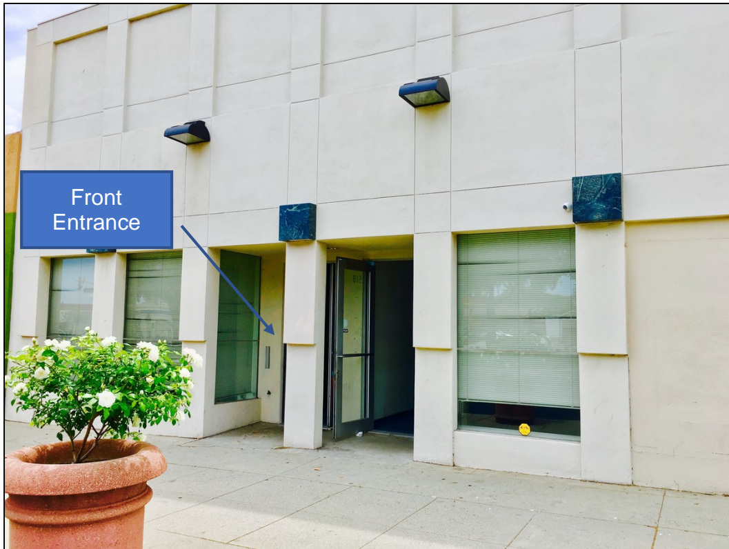
Front Entrance – View looking west from Euclid Avenue
