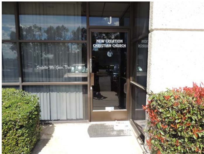
Existing Unit J - Front Entrance
