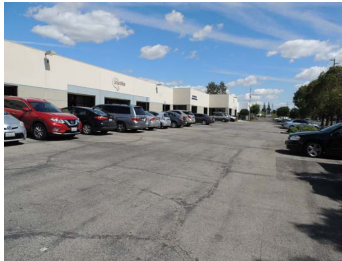
Southeast View of Existing Building & Parking Area
