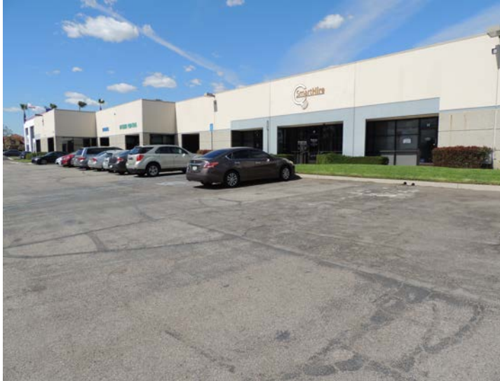
Southwest View of Existing Building
