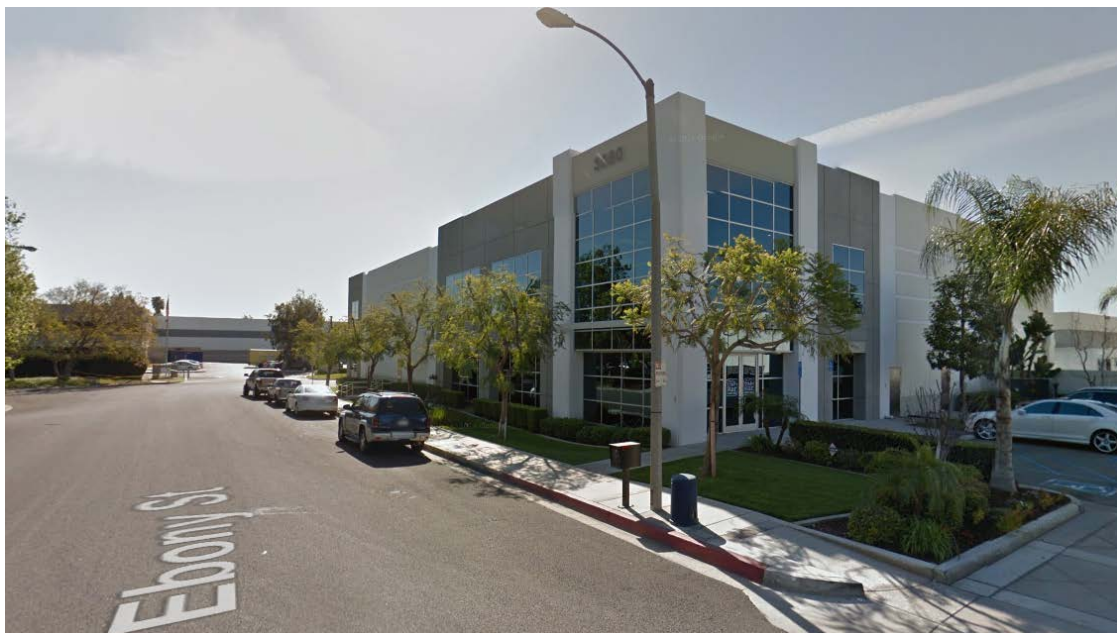
VIEW LOOKING SOUTHEAST FROM EBONY STREET
