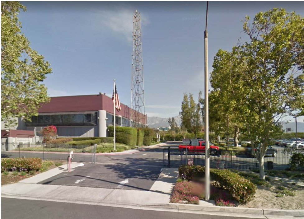
NORTHEAST VIEW OF THE BUILDING FROM EBONY STREET
