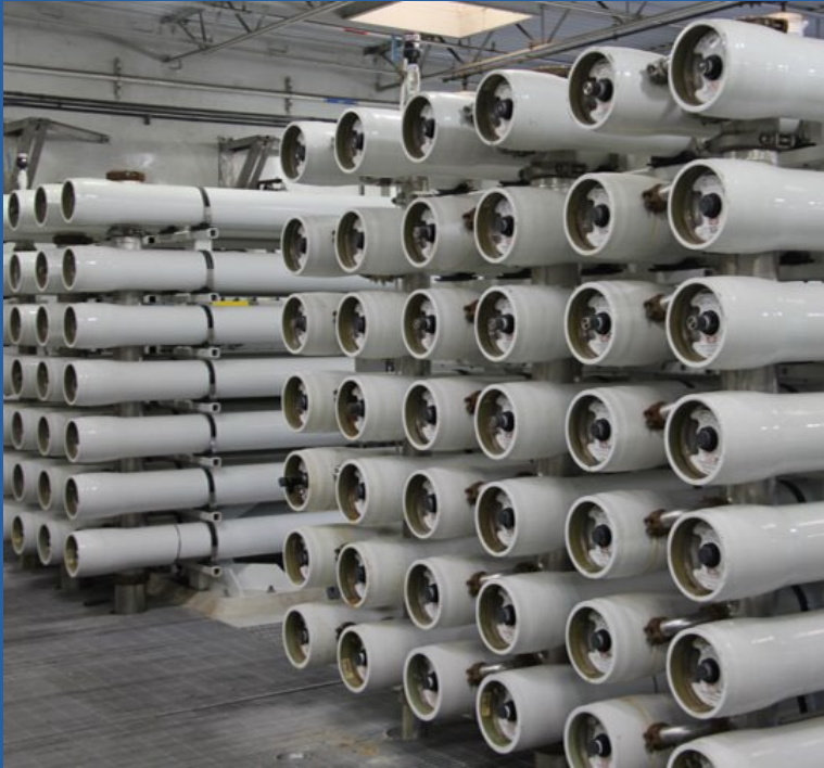
Stainless Steel Tubes Used in Reverse Osmosis System, c. 2000s Digital print Courtesy of the Inland Empire Utilities Agency
