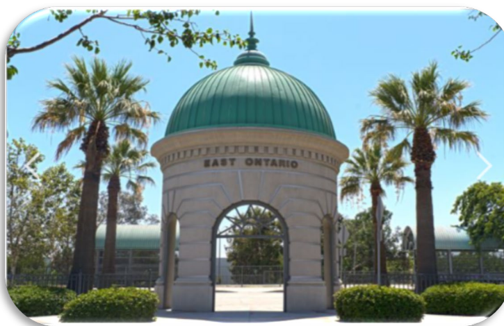
Metrolink's East Ontario Station, located in the City of Ontario. Photo Courtesy of Metrolink
