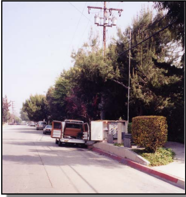
Figure 5-6 – Magnolia Pump Station
