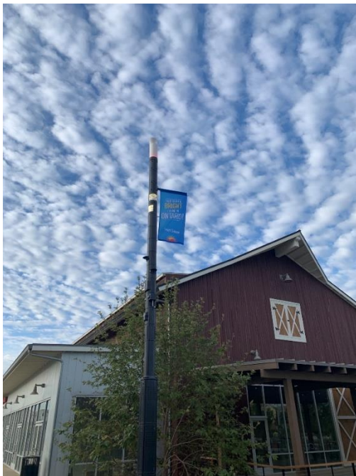
ENE HUB station at New Haven Marketplace – street furniture that provides lighting, phone charging, wifi and 5G service, wayfinding, security and even speakers for streaming music or announcements. Photo by Brookfield Residential.
