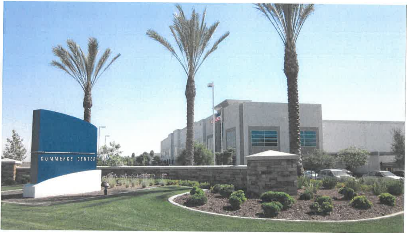
Photo 7.3 - Example of Industrial building
