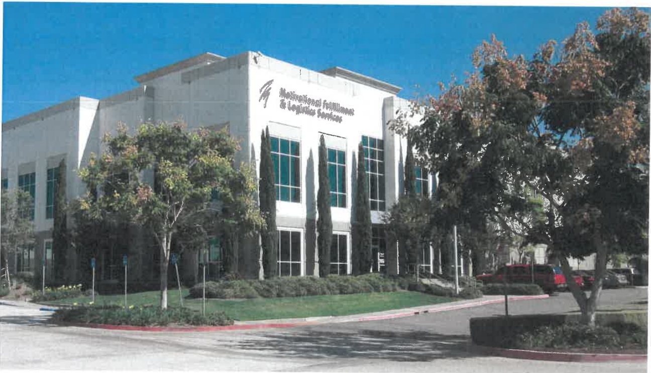
Photo 7.2 - Example of Industrial building
