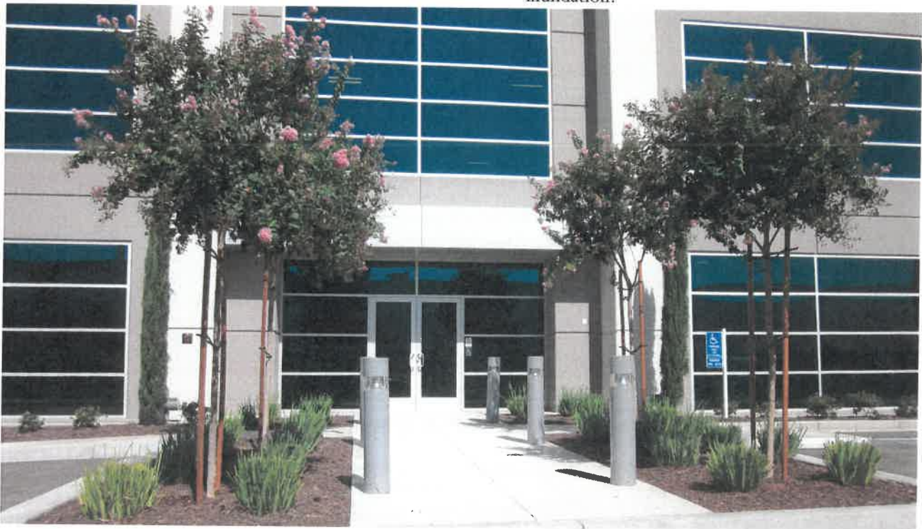
Photo 7.5 - Example of Industrial lighting at office entry
