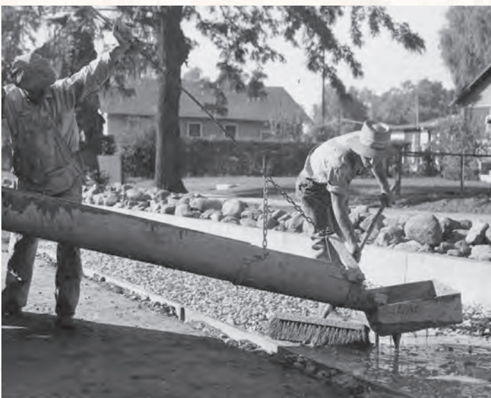
Street Improvements on Euclid Avenue
