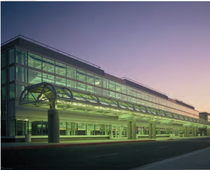
LA/Ontario International Twin Terminals
