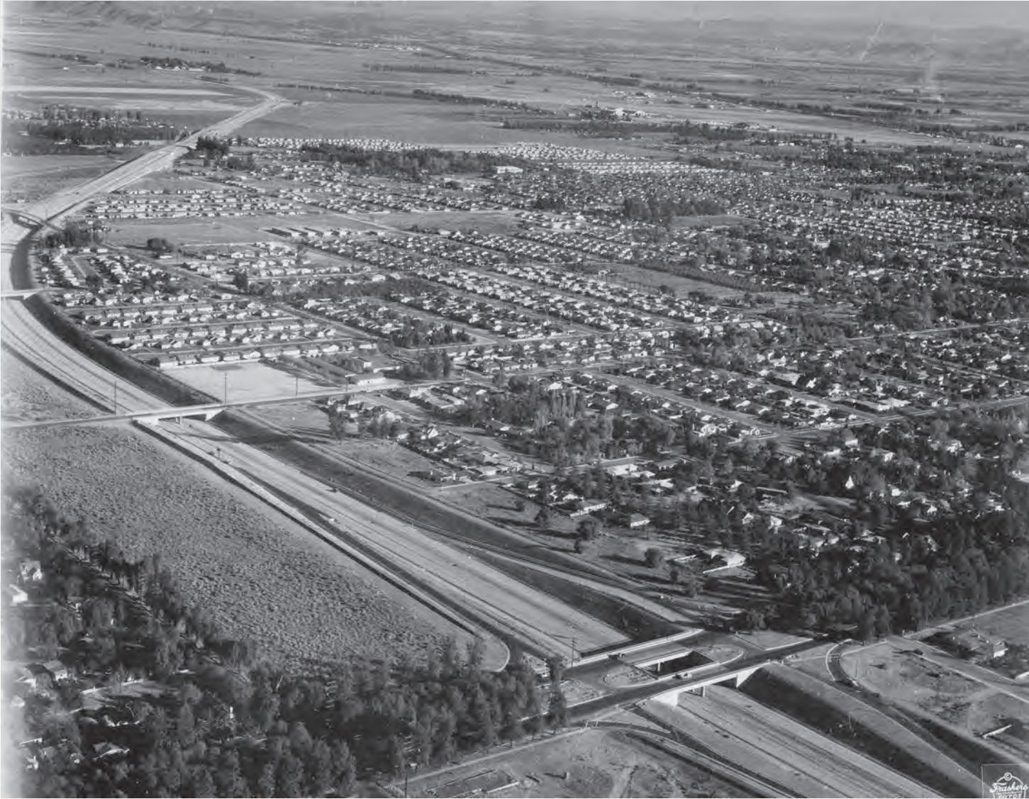
San Bernardino Freeway (I-10) at the Euclid Avenue Bridge and Interchange
